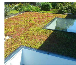
sedum blanket green flat roof and roof lights
