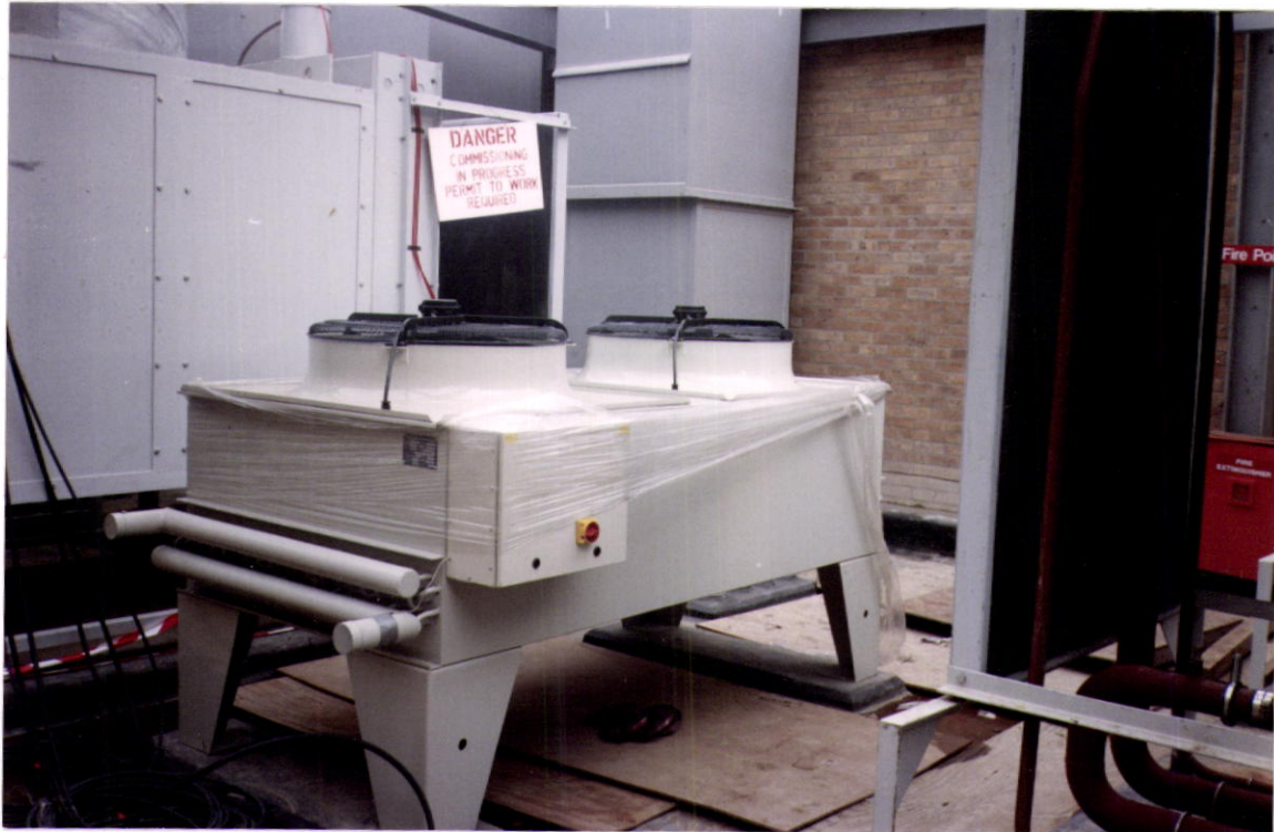
COLOUR PHOTOGRAPH OF GENERATOR.
