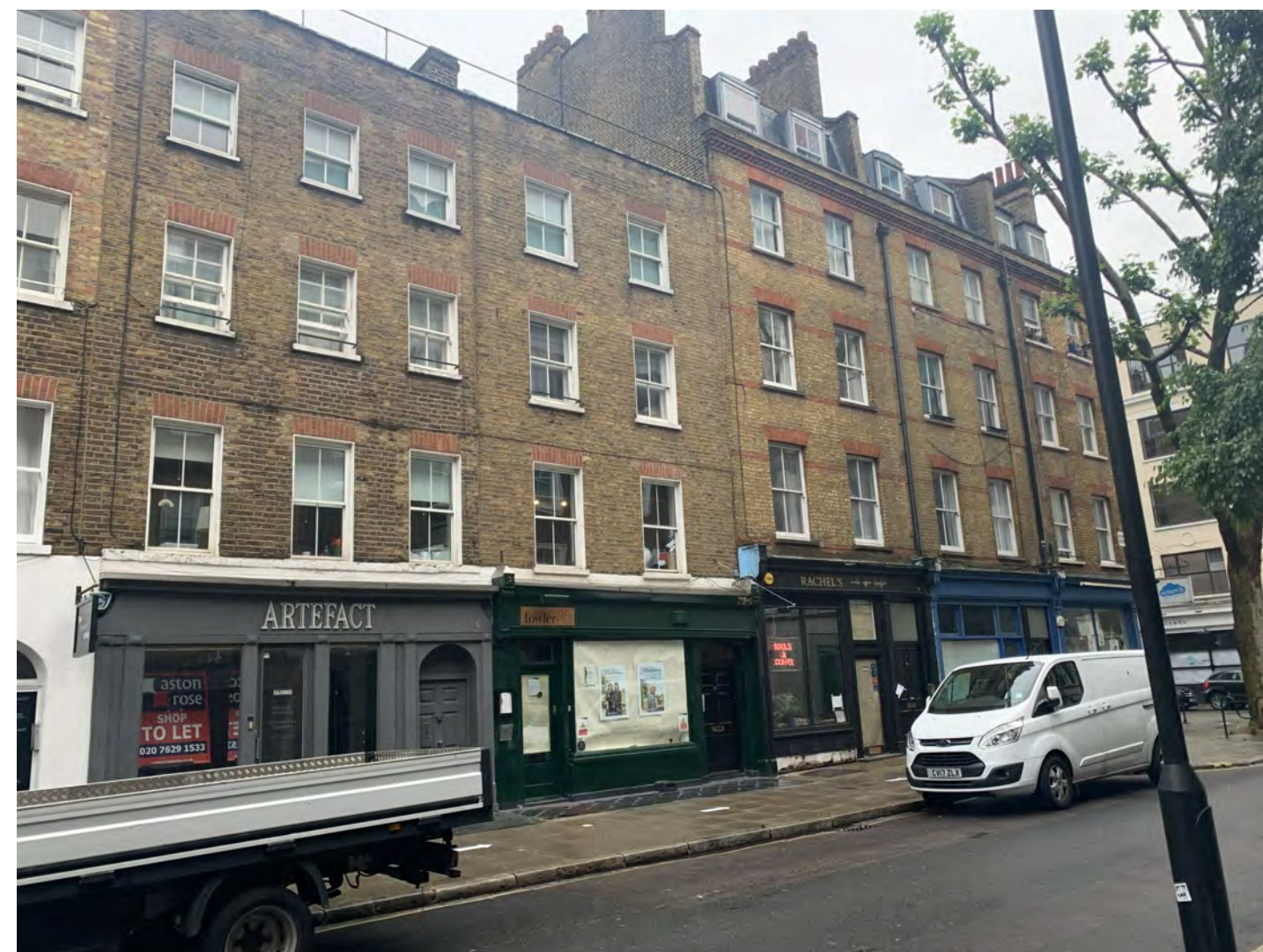
View facing north east showing front of 32-36 Windmill Street
