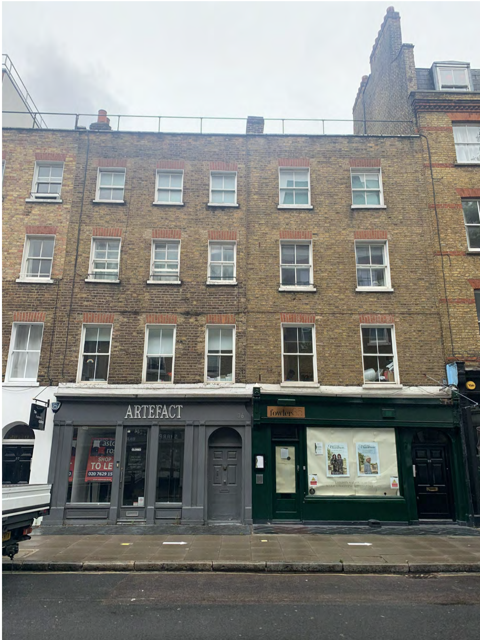
View facing north west showing front of 35-36 Windmill Street
