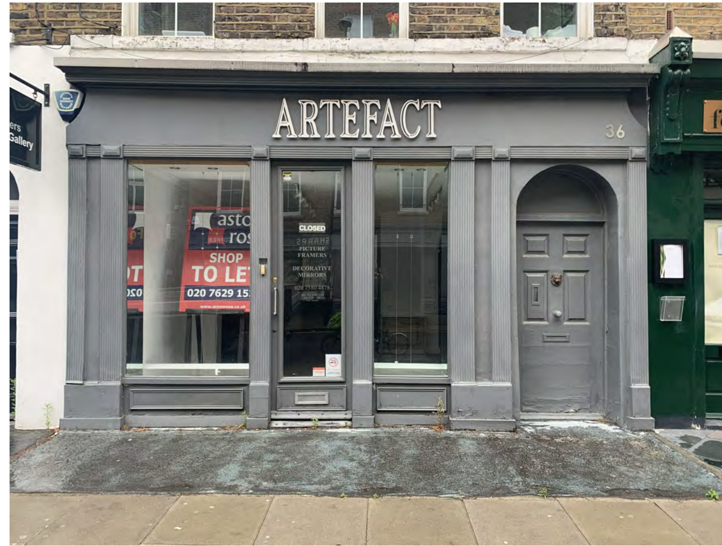
View showing existing 36 Windmill Street shopfront
