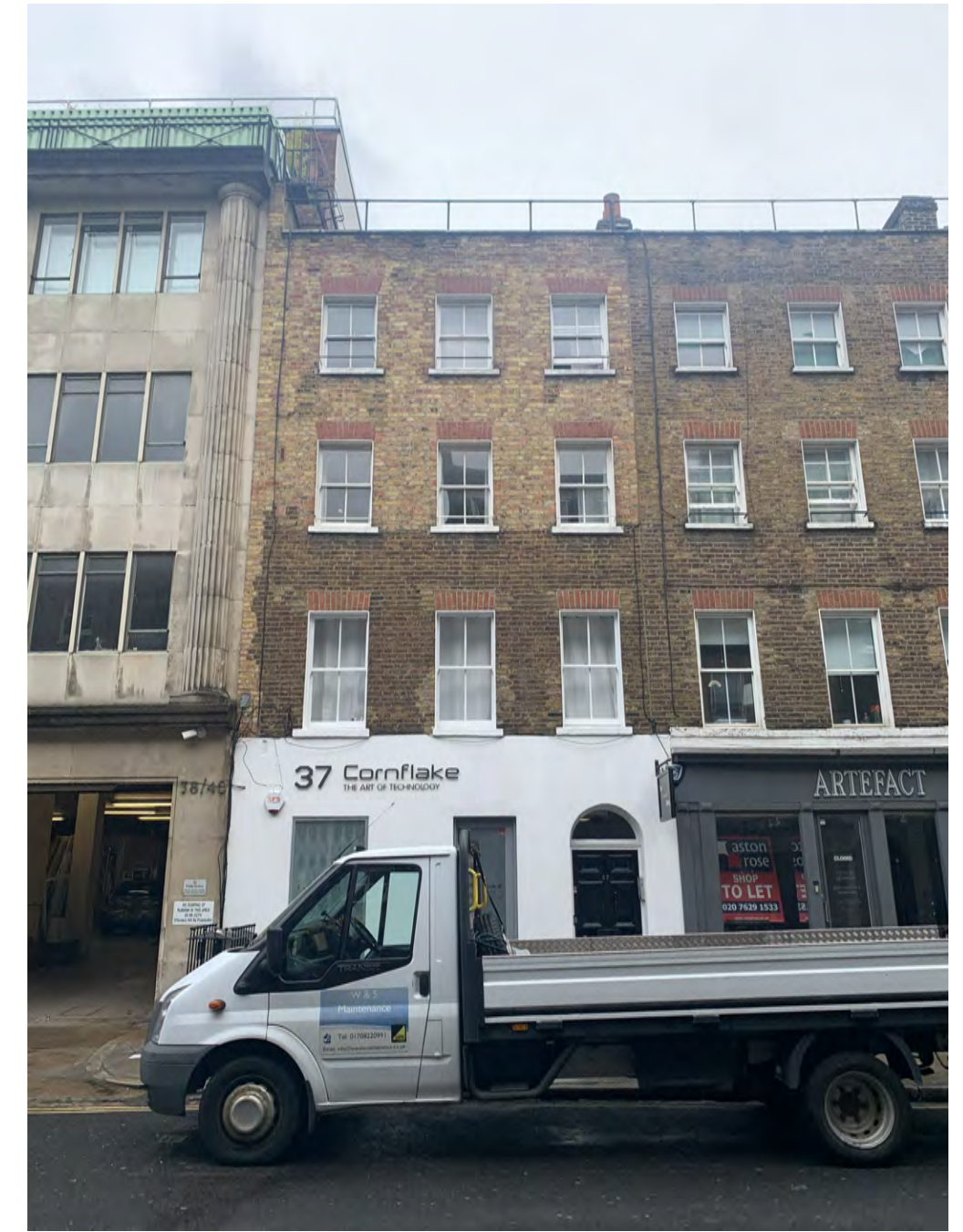
View showing existing 37 Windmill Street shopfront
