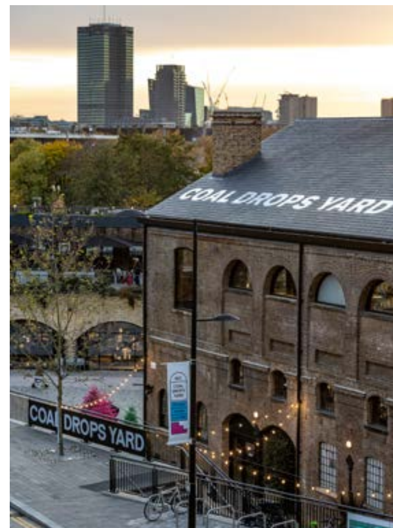
Figure 4: Temporary signage on the Eastern Coal Drops, visible at dusk.
