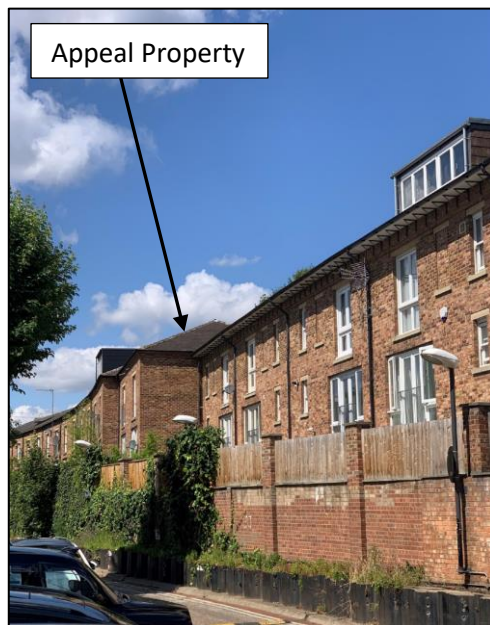
Existing View of No. 25 Facing West
