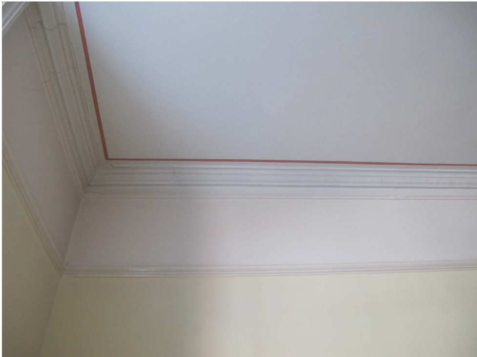
Fig. 5.3 Existing picture rail and cornice
