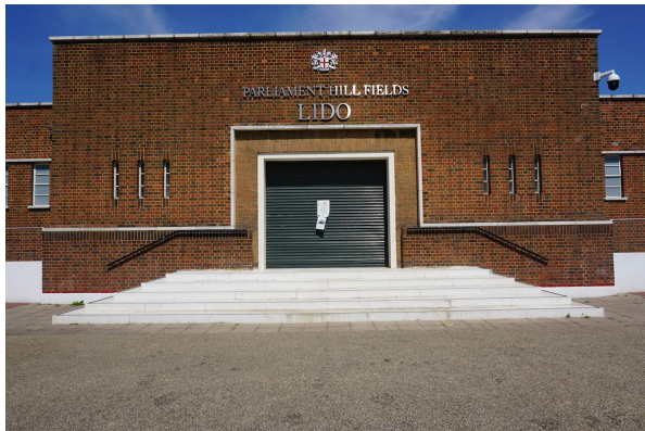
The symmetrical façade and restrained modernity is characteristic of the best LCC work of the period
