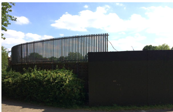
The pre-2016 fence prior to collapse
