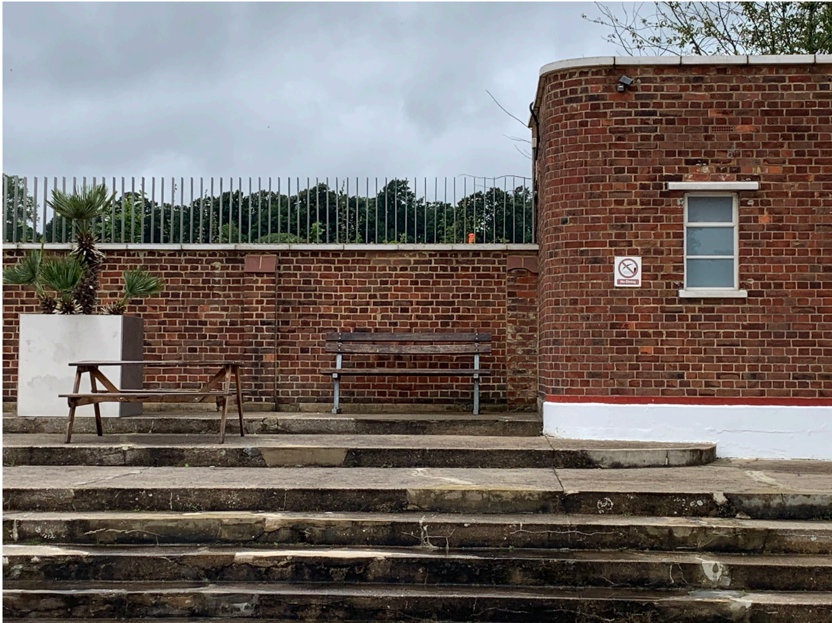
Photos taken from inside the lido looking north towards the rear wall. The post, with red tape, is 2.4 metres in height at the tip (i.e. max height of proposed fence).
