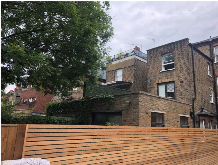
View of similar roof terrace along the terrace
