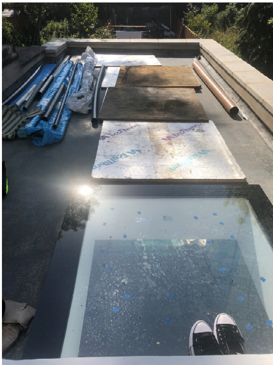
View of existing roof as built ahead of making this application.
