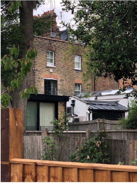
View of similar roof terrace along the terrace
