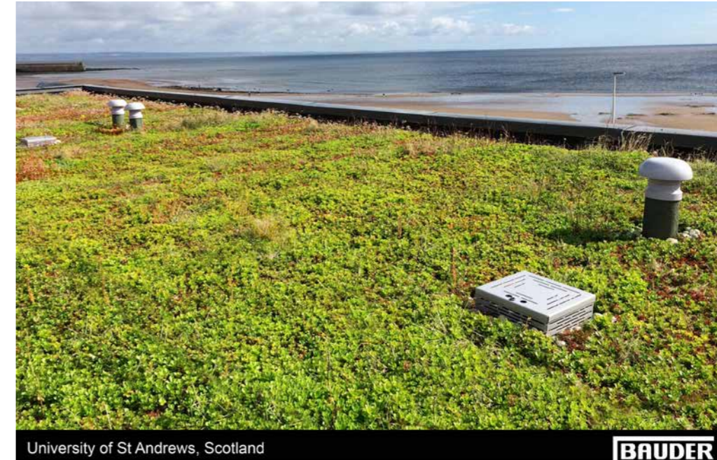
Reference of Bauder sedum blanket green roof. University of St Andrews, Scotland
