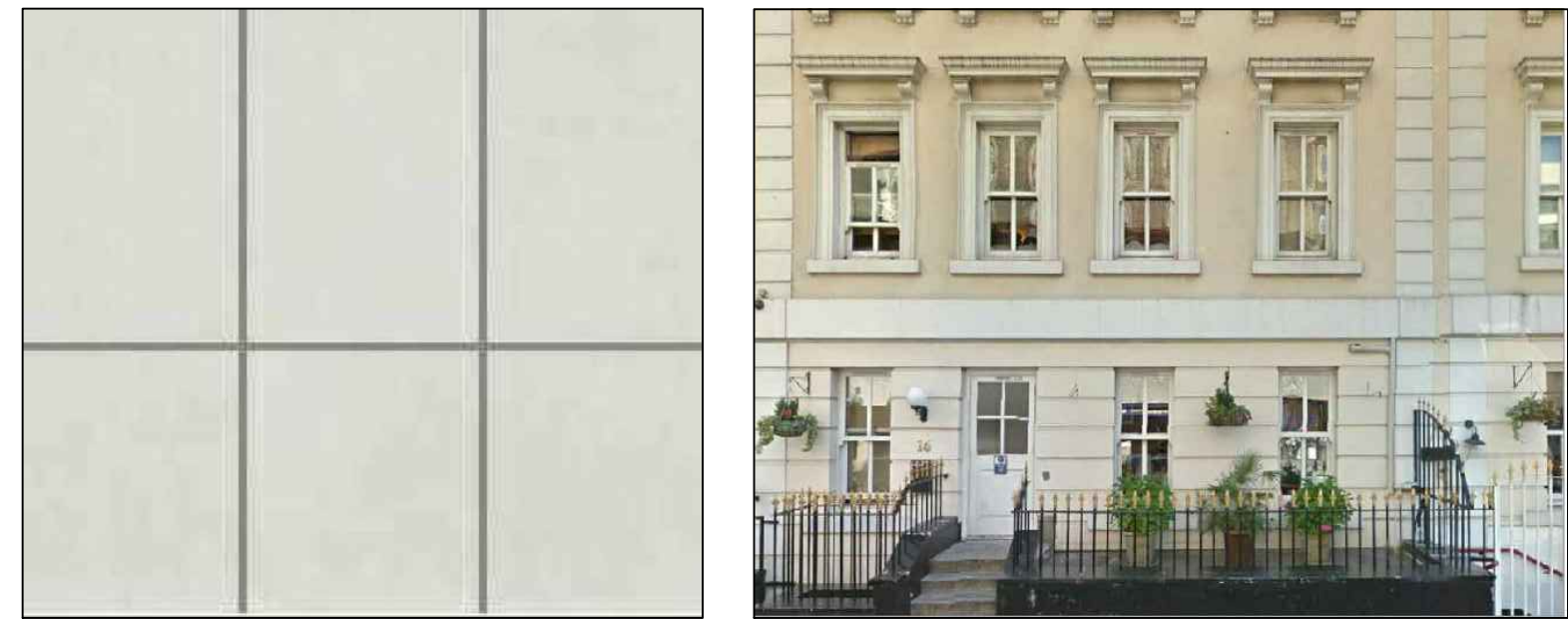
Fibre cement cladding to be used to mirror the proportion of the banding on the facade of the hotel building opposite, with a similar colour used.
