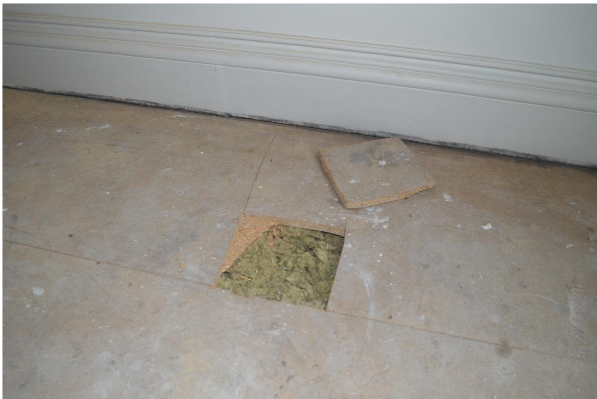
First floor front room- chipboard. No boards retained beneath.
