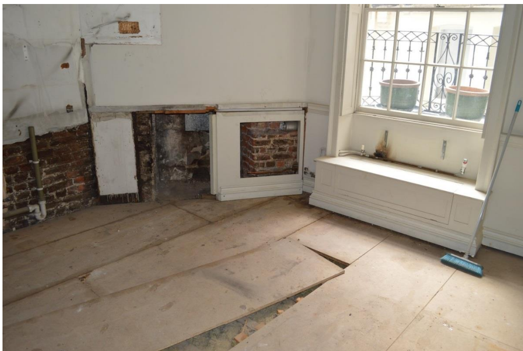
First floor kitchen – whole room is chipboard. No boards retained beneath.
