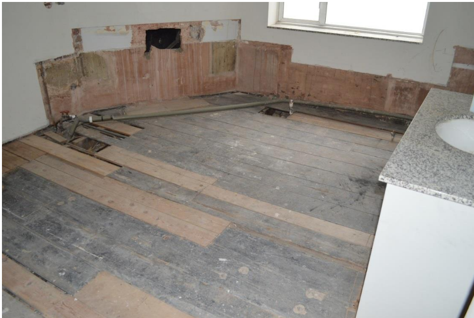
Third floor bathroom – a few possibly original boards but mixed with modern boards and 19 th or 20 th century boards.
