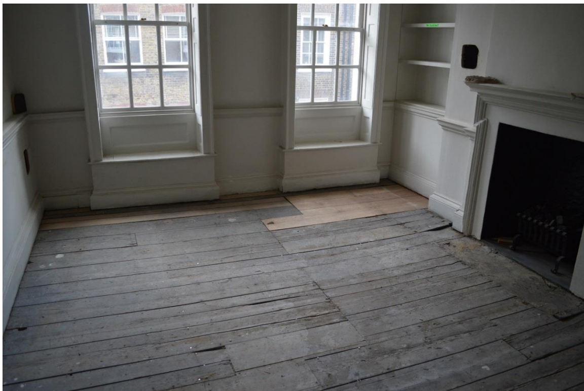
Second floor front room - possibly original Georgian boards but in poor condition. A small section of modern boards towards the windows on the front elevation.
