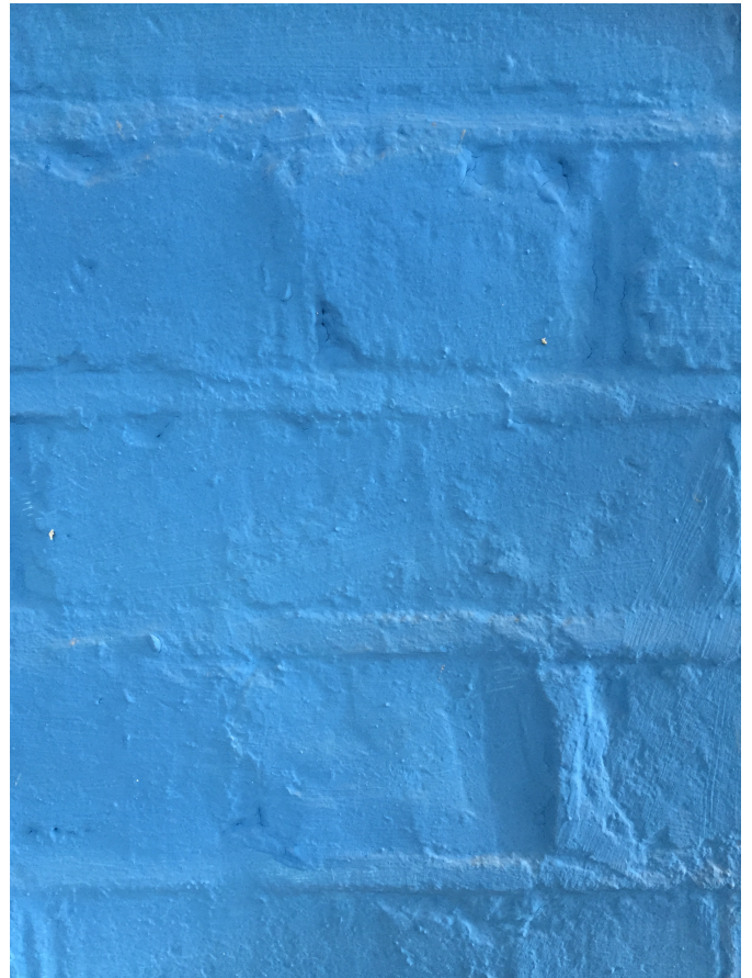
Sample blue paint applied to brickwork on 82 Neal Street
