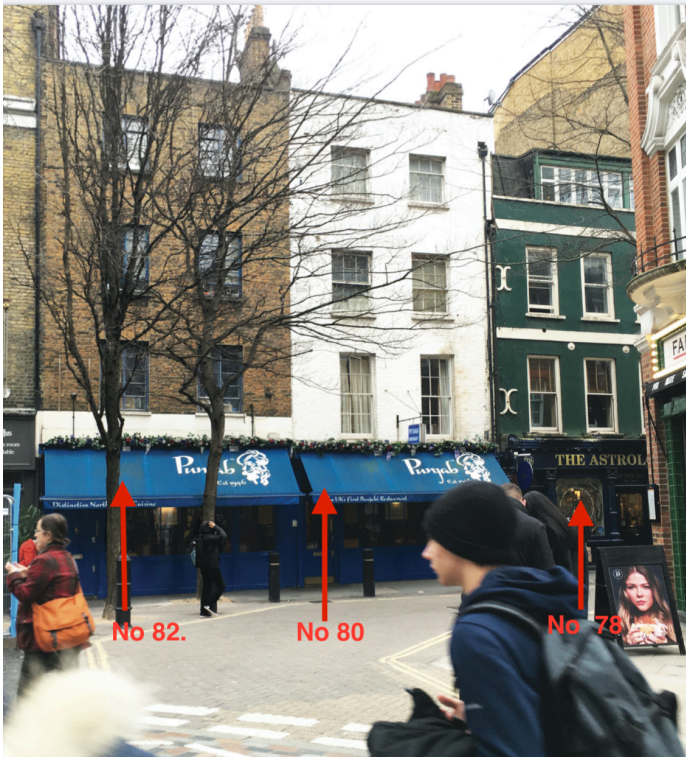
Front elevation : Photograph taken in 2015. No 78 and No 80 are both listed Grade II
