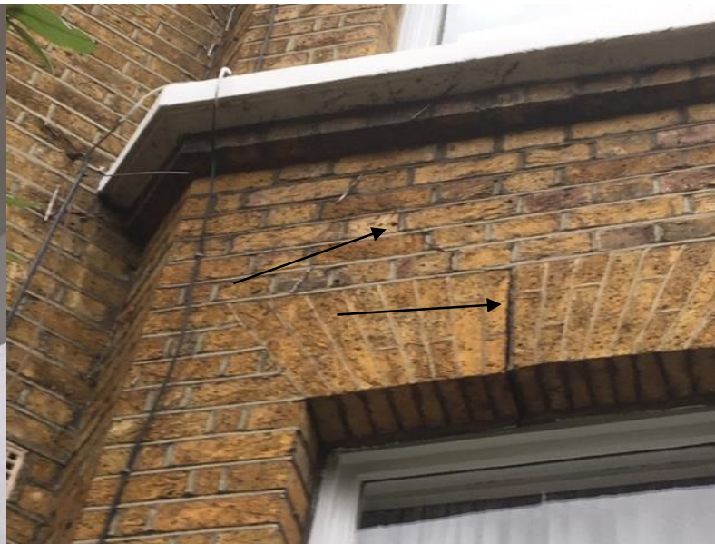
Cracking to bay
