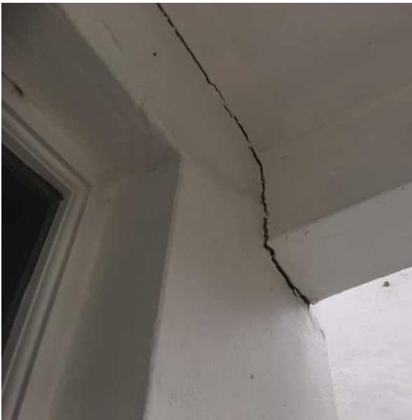
Cracking to porch
