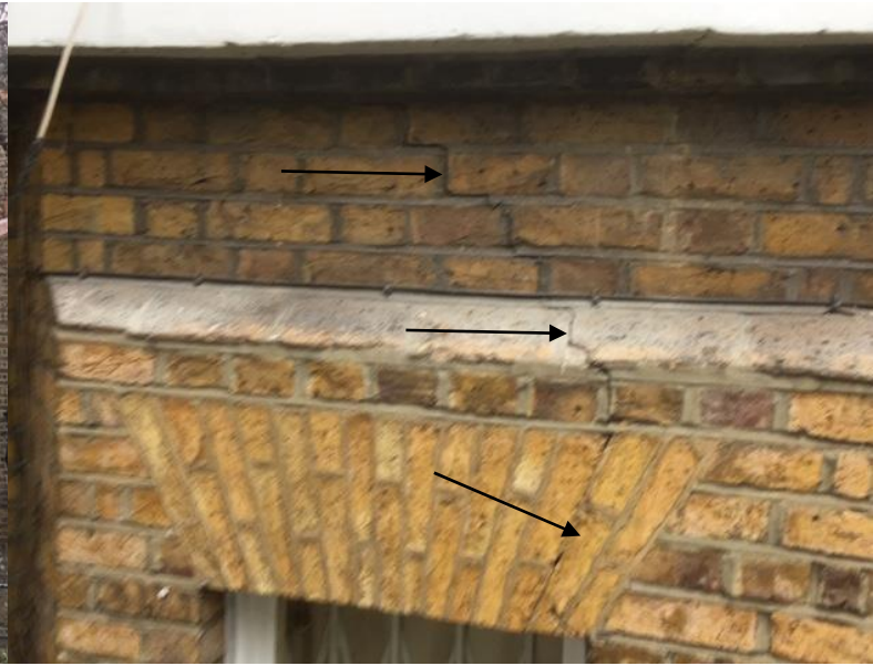
Cracking to bay
