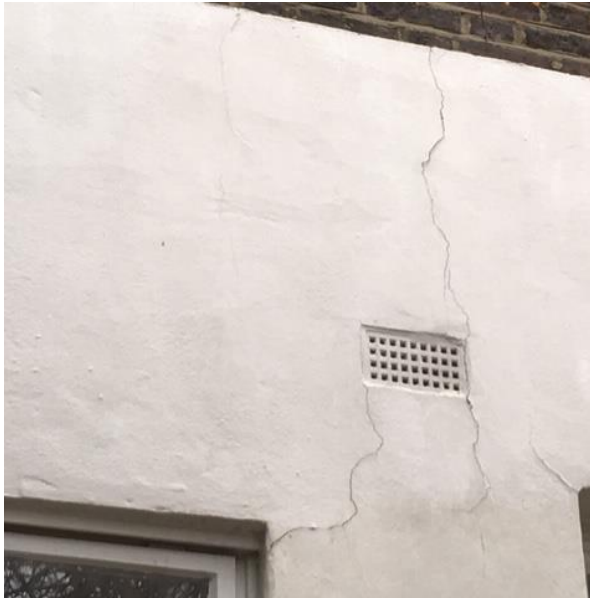
Cracking to rear elevation
