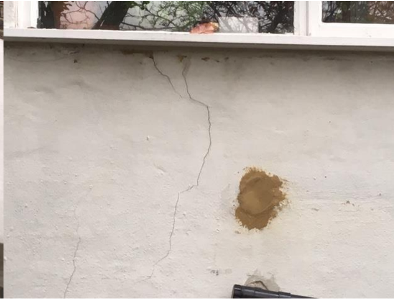
Cracking to rear elevation
