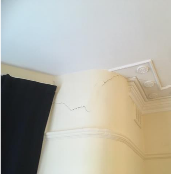
Cracking to first floor flat
