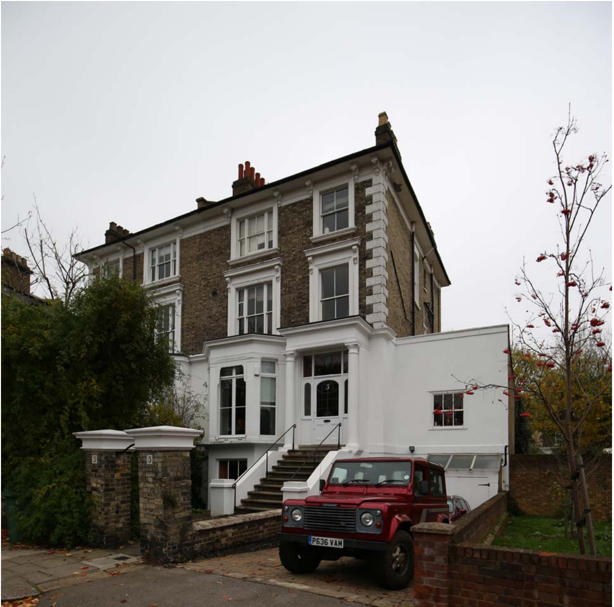
View of the existing front elevation
