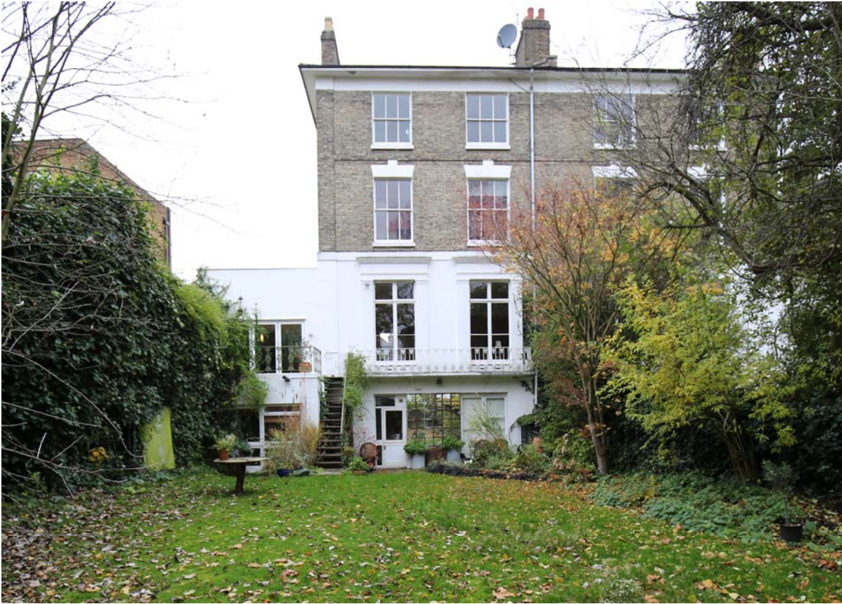
View of the existing rear elevation
