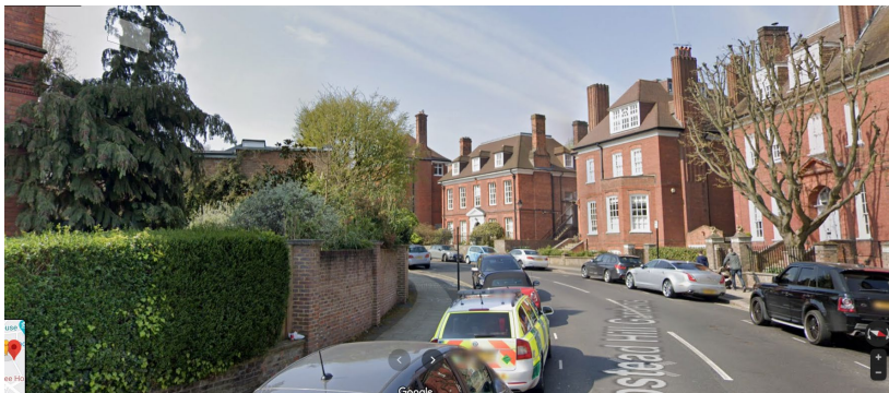
Current view west, turning the curve in the road to the group of Grade II listed buildings – 4B hardly visible on the left. (Image source: Google Street view, accessed July 9 th , 2020)
