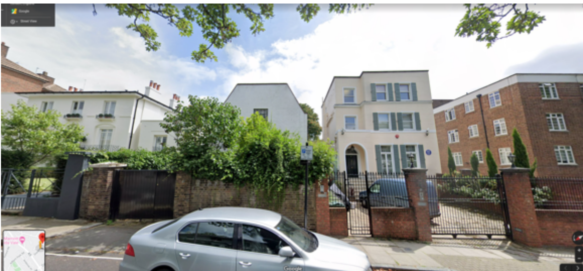
An example of the street elevation showing the variety of property types in the road, some later conversions have created properties that do not fit into the typology of the area. Many properties have certainly not been preserved in the style as they would have been built in 1820s, and so the street is a mismatch of styles and is not a good representation of the oldest part of the Conservation Area.
