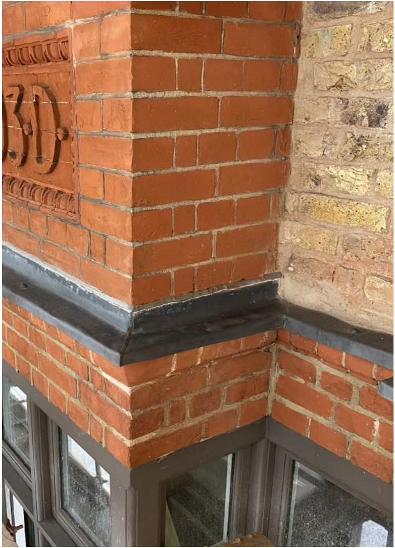
Close-up detail showing repaired brickwork and lead flashings Red rubber brickwork has been carefully repaired and cleaned - lead flashings installed to projecting brickwork to protect leading edges which are soft and liable to erosion
