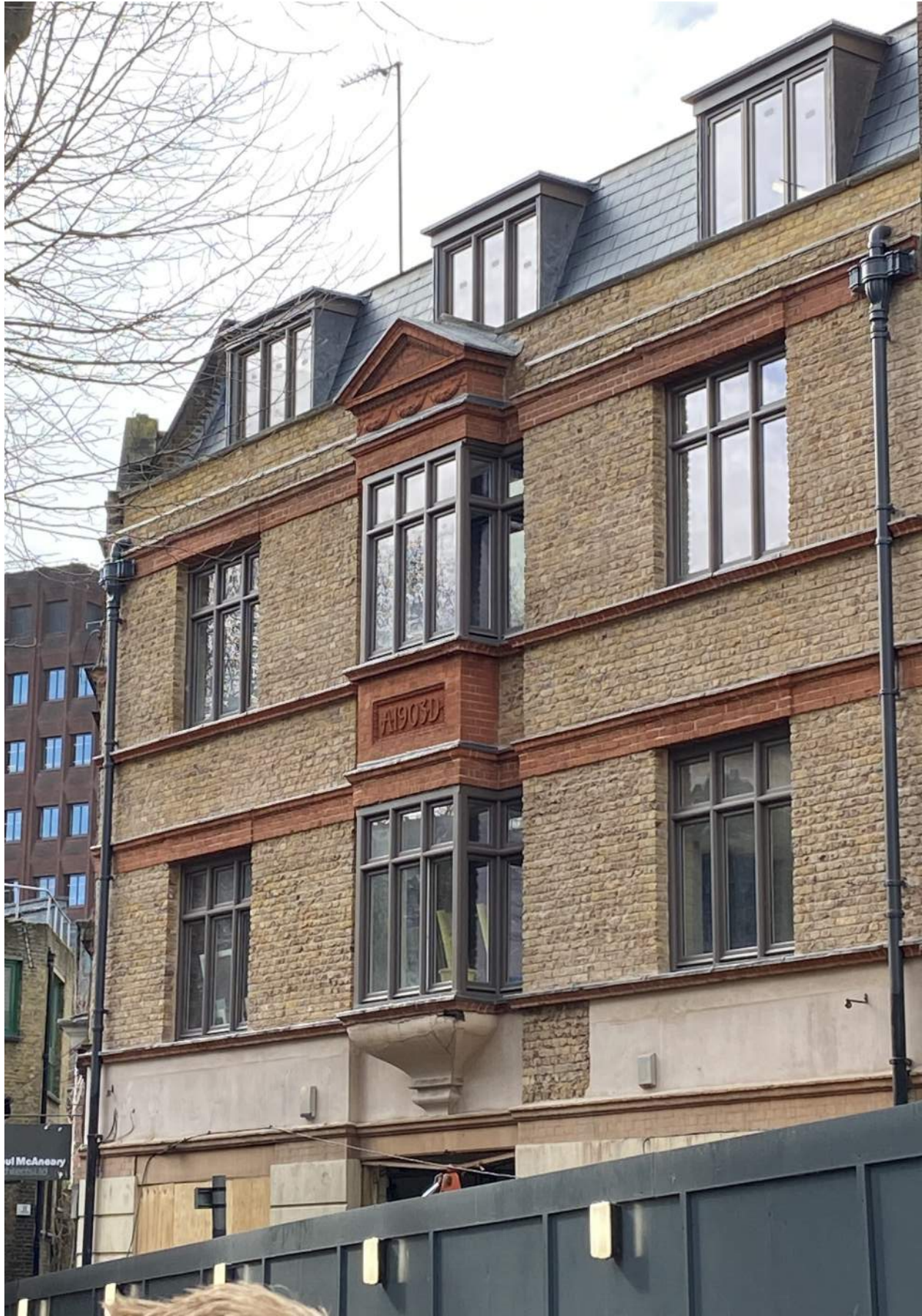
4 Flitcroft Street - front facade showing render removed to First and Second Floors - existing stock brick revealed beneath - bricks have been carefully cleaned and repaired by hand creating a soft consistent appearance.
