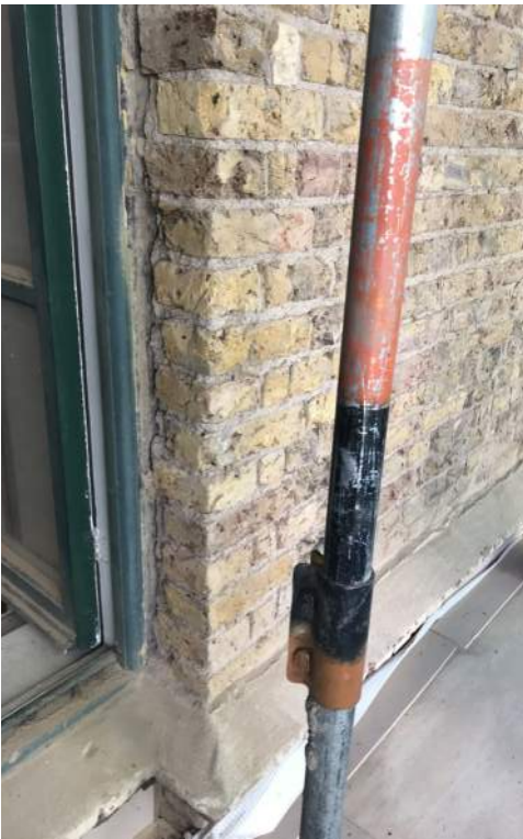
Close-up detail showing render removed - existing stock brick revealed beneath - generally in good condition with light surface damage due to later applied render but brick integrity largely intact. Areas/Bricks with significant damage to be made good in matching brick where the removal has resulted in the loss of the brick surface and would compromise weatherproofing/façade integrity. Mortar joints to be repointed where required
