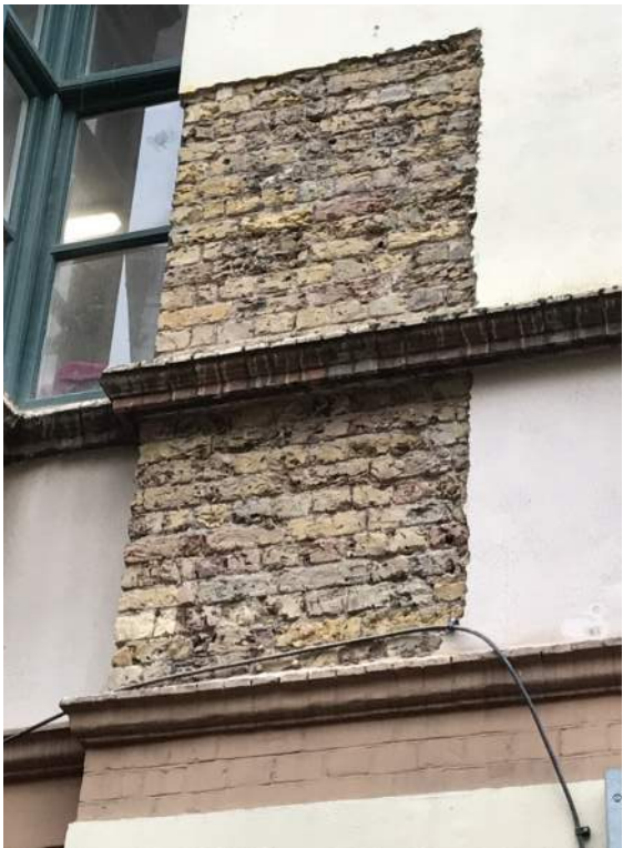
Close-up detail showing render removed - existing stock brick revealed beneath - generally in good condition with light surface damage due to later applied render but brick integrity largely intact. Areas/Bricks with significant damage to be made good in matching brick where the removal has resulted in the loss of the brick surface and would compromise weatherproofing/façade integrity. Mortar joints to be repointed where required
