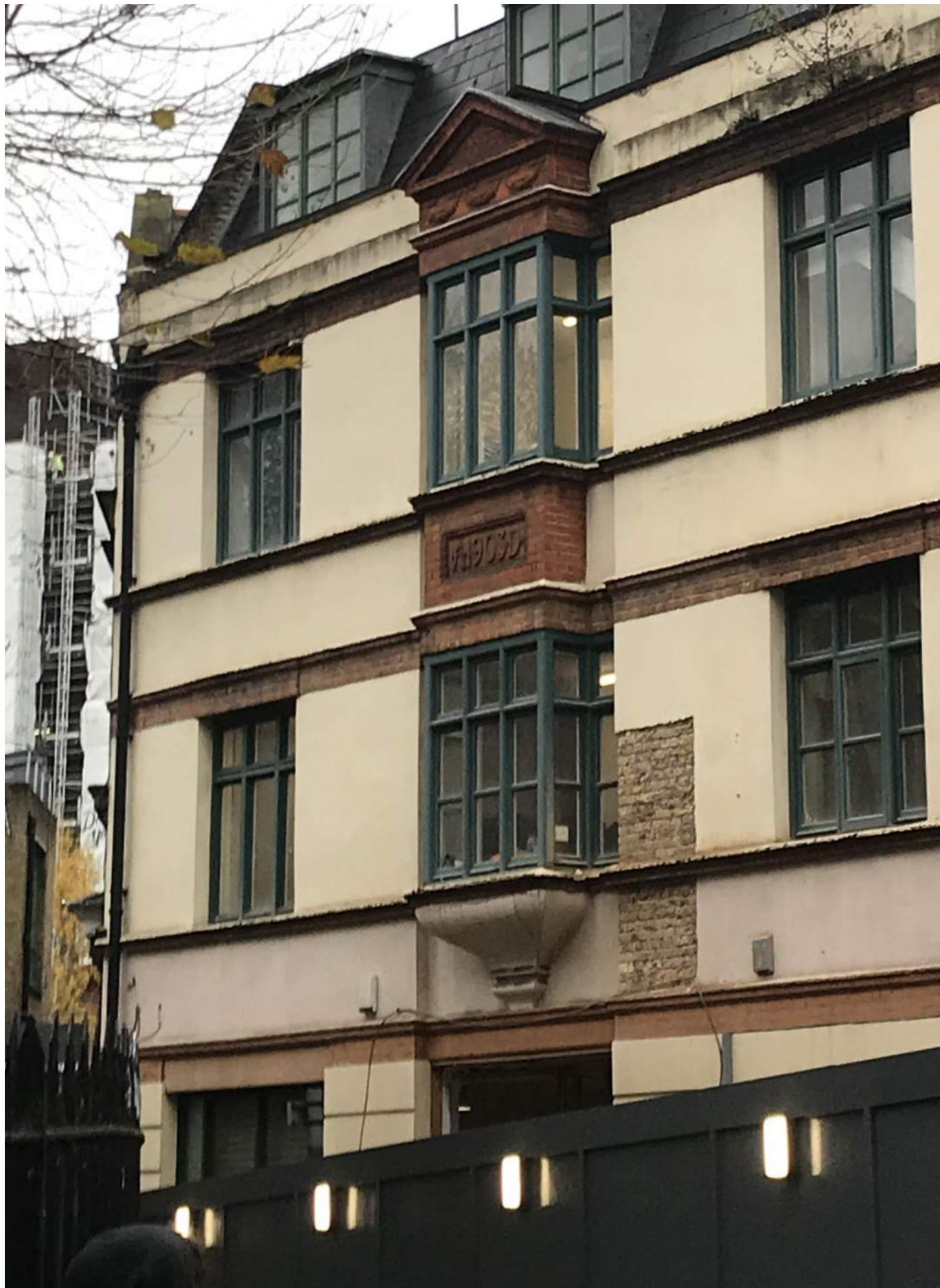
4 Flitcroft Street - front facade showing render removed to First Floor sample area - existing stock brick revealed beneath - generally in good condition with light surface damage due to later applied render but brick integrity largely intact.
