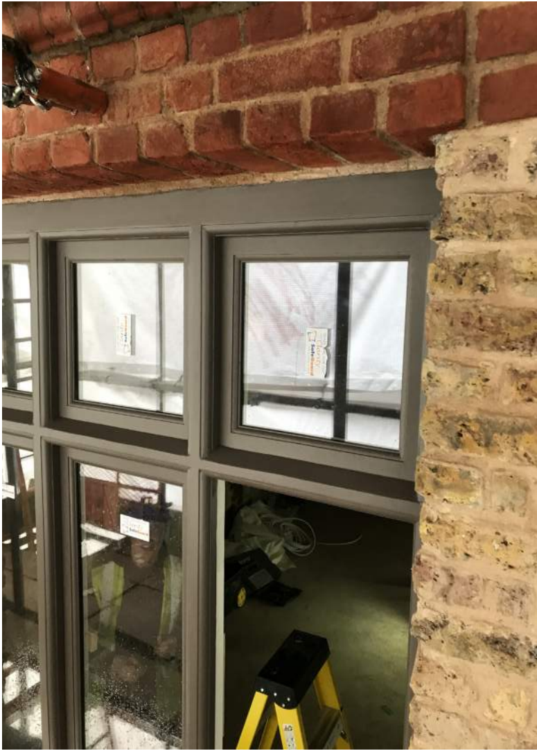
Close-up detail showing render removed - Existing bricks have been revealed showing historic surface damage to the fired-face - this is the result of scratching to create a key for the render when originally applied. The bricks are generally in a good condition and any that have had deeper breakage/damage have been replaced with matching stocks. Pointing has been repaired in lime mortar - the pointing has been slightly recessed to allow the reading of the brick edges to be maintained and keep the mortar joints. A delta membrane is provided internally to mitigate any dampness
