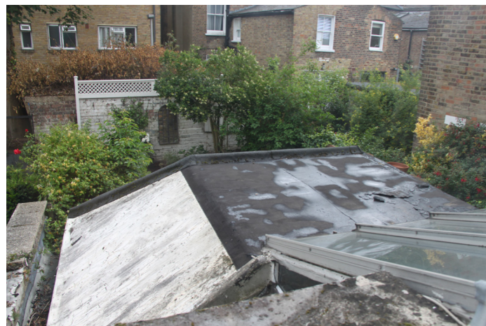
EXISTING EXTENSION ROOF
