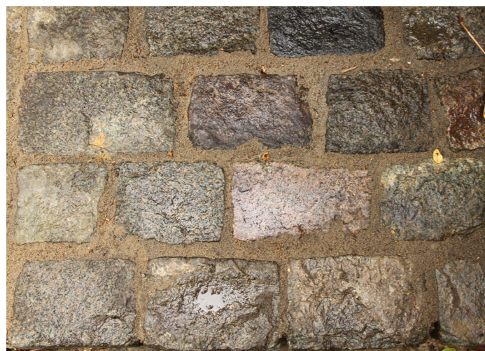
EXISTING GRANITE SETTS IN REAR COURTYARD
