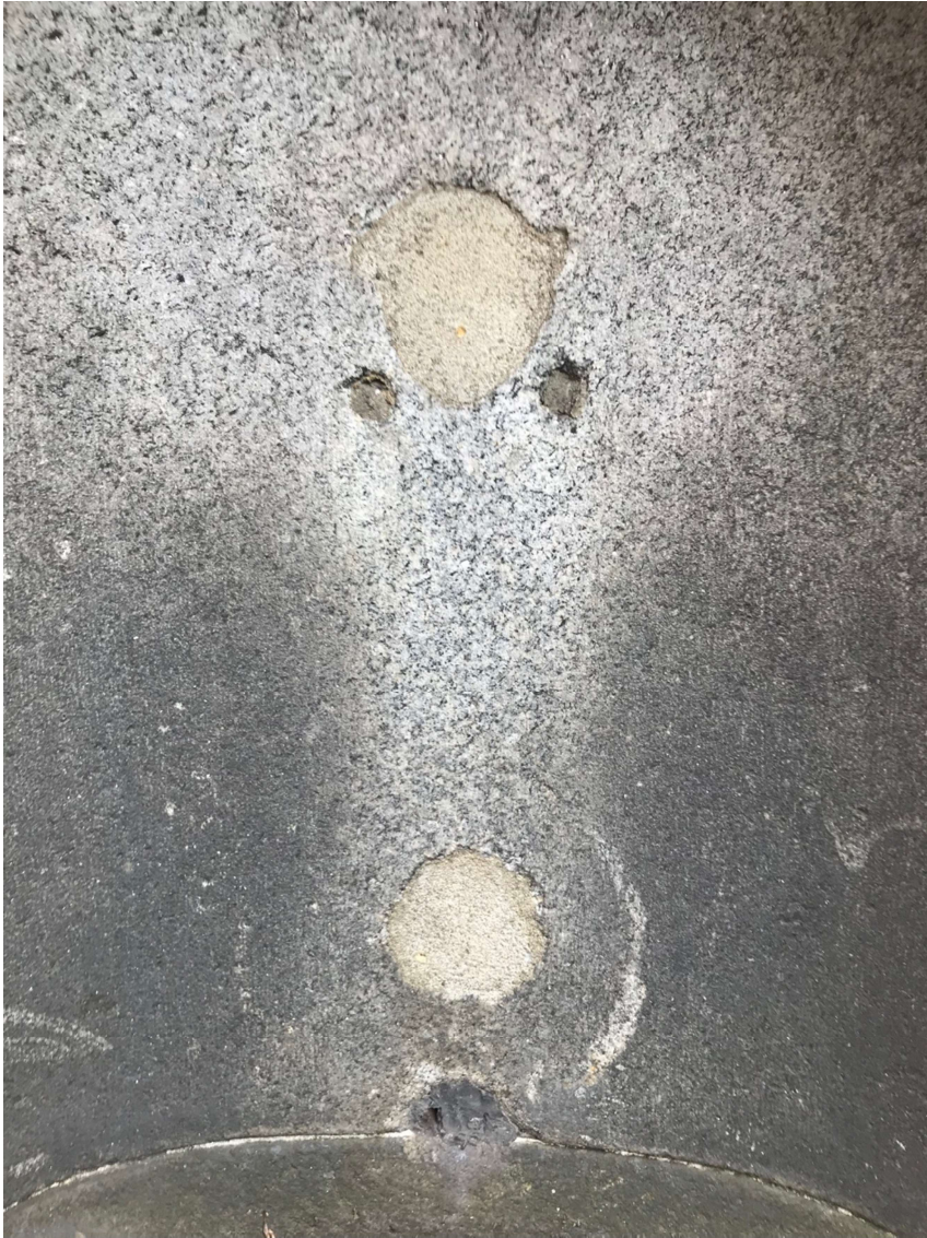
Cement repairs where faucet removed
