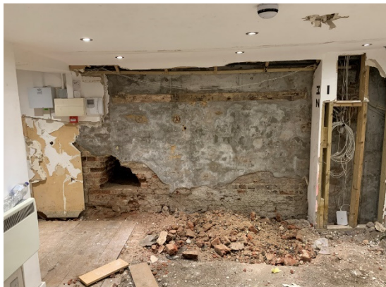
Figure 6 Holes opened in flank wall into gap
