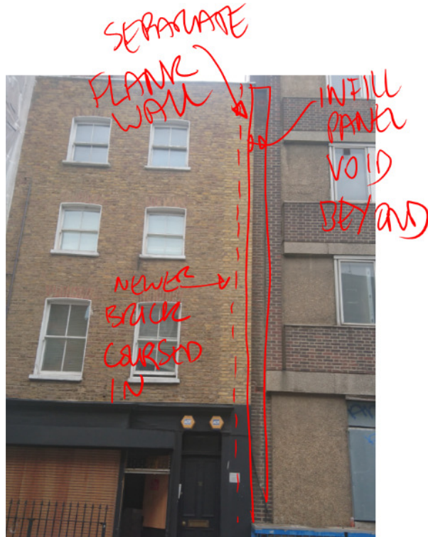
Figure 2 Existing street elevation east boundary
