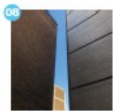
08 Small gap between the site's rear wall on the left and Arthur Stanley House on the right
