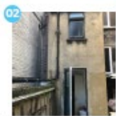
02 View of back elevation, from above the ground floor extension
