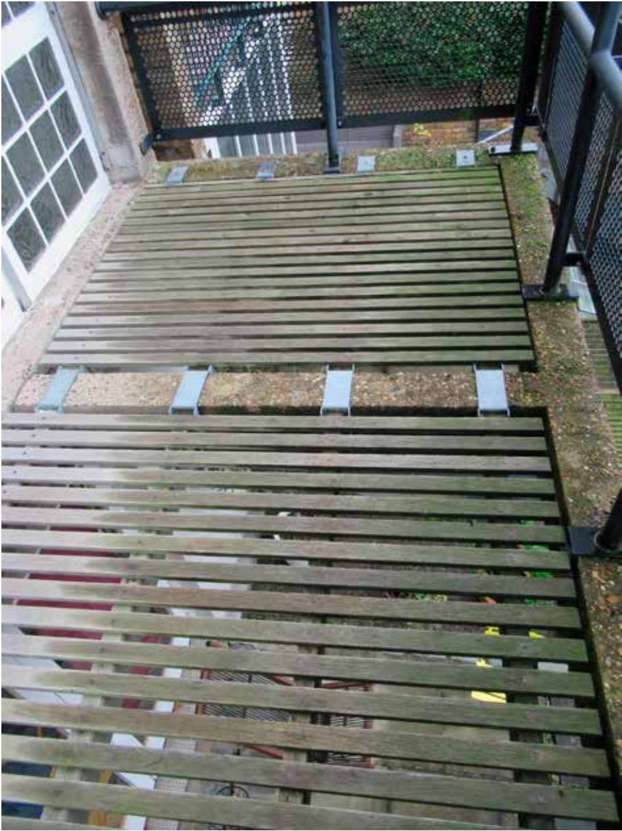
Fig. 3.11: Timber decking on rear balcony in need of replacement.
