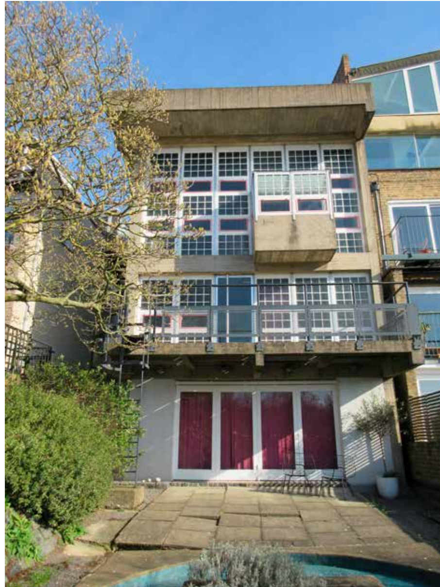
Fig. 3.3: View of rear facade from the garden, showing the later, added timber bi-fold doors at lower ground level, and the balcony with timber decking at ground floor level.
