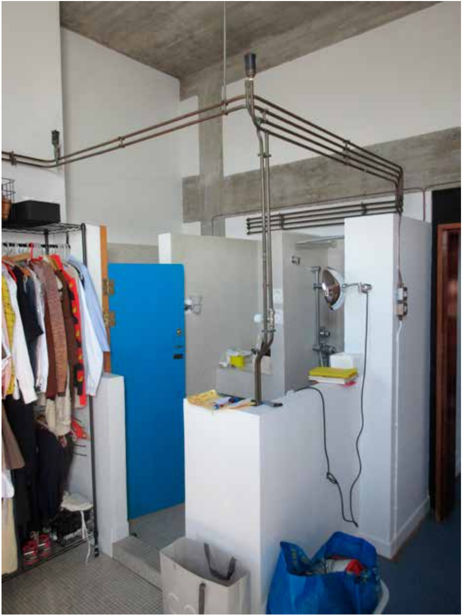
Fig. 3.13: Ensuite bathroom in the master bedroom with central heating pipes threaded through the space, first floor.
