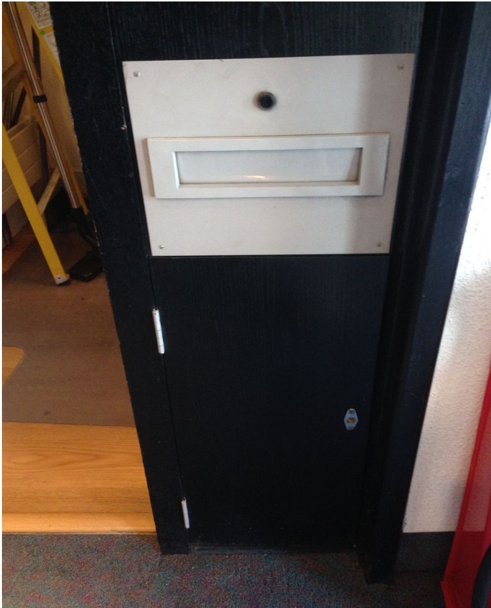
Photograph 4: Typical plating adjacent to letterbox
