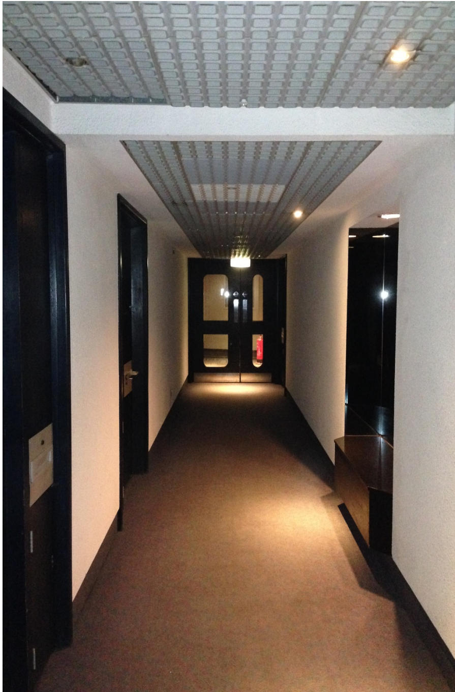
Photograph 5: View of part of a typical communal corridor showing the flat front entrance doorsets located on either side. The corridors form part the protected means of emergency escape route for residents from Centre Point House.
