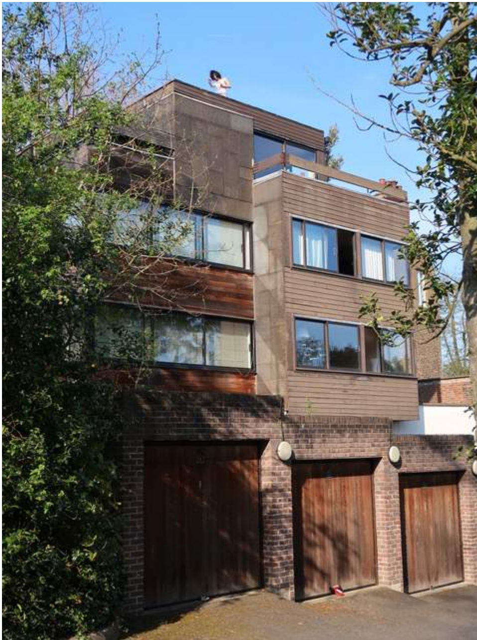
photo of mock-up of glass balustrade as it would appear from south side
