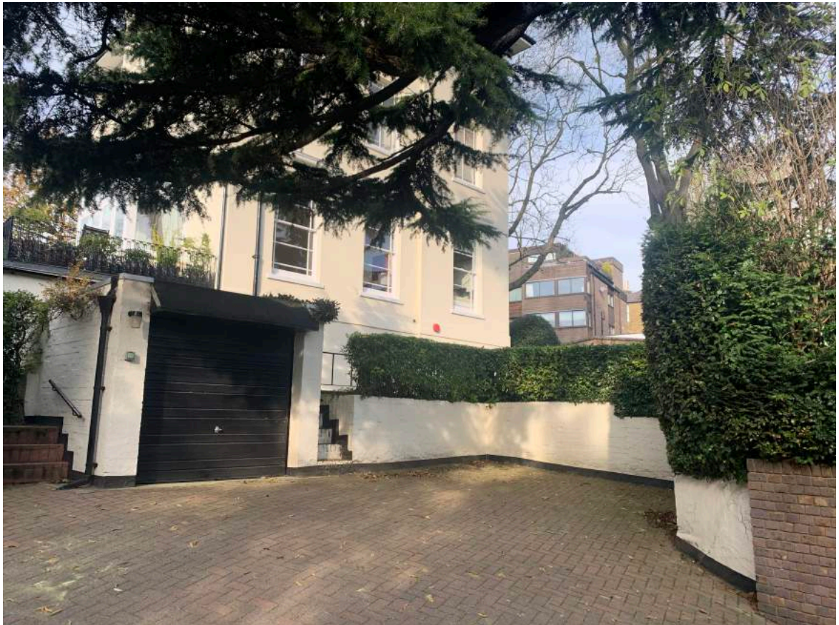
South East Elevation from 1 Oak Hill Park Mews
