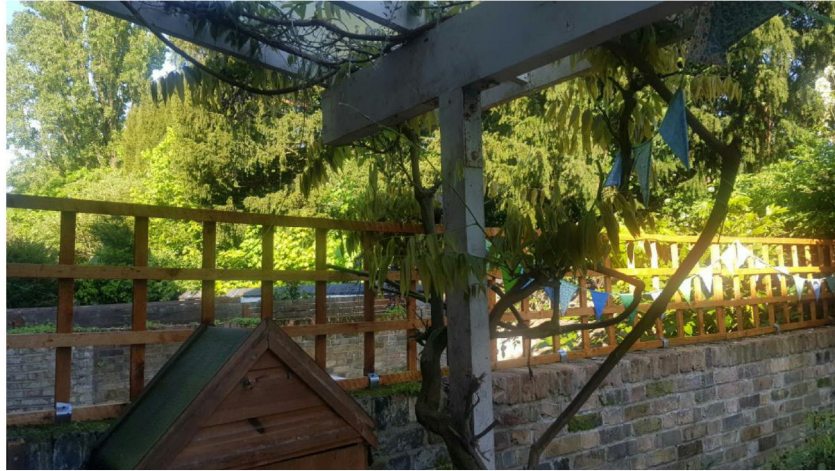
View from rear wall of no. 70 looking towards application site.
