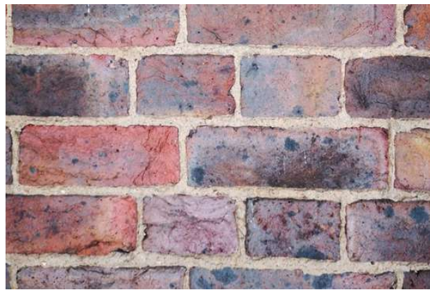
01 Flemish bond dark multi-stock brick to external facade
