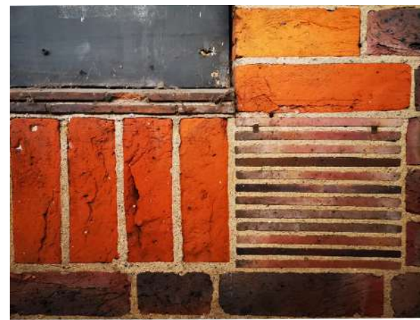
04 Creasing tile to window corners Soldier course window heads and sills
