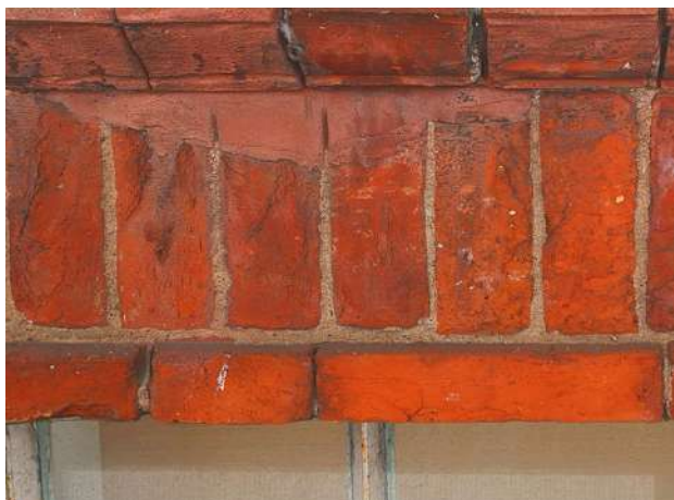
03 Brick banding Soldier Course and special sill brick band
