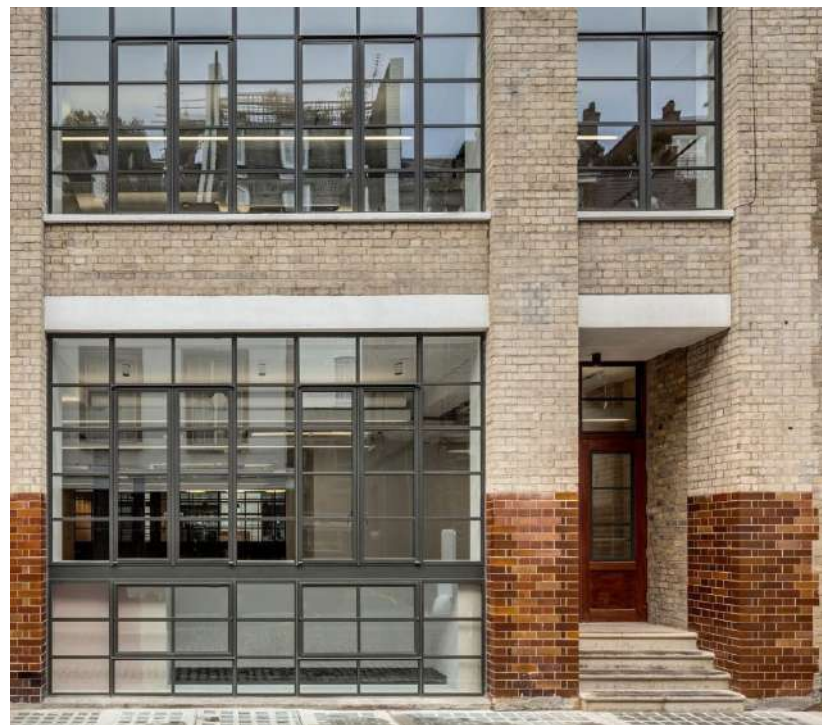
Crittall windows have slim glazing bars and are beaded in the traditional manner - (116 Marylebone Lane - Morrow+Lorraine)
