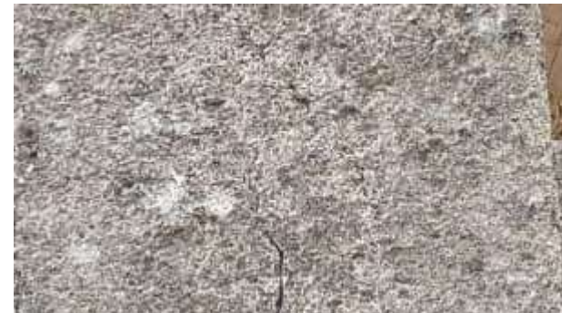
Photographs of the existing coping, decorative scroll and window surround showing the cast concrete and stucco render has become damaged and pitted.
