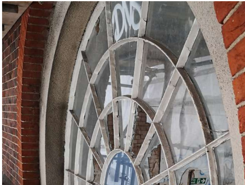
Photographs of the existing coping, decorative scroll and window surround showing the cast concrete and stucco render has become damaged and pitted.
