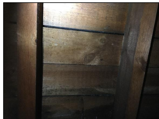
Figure 5: BRM lining and close board panelling of roof void
