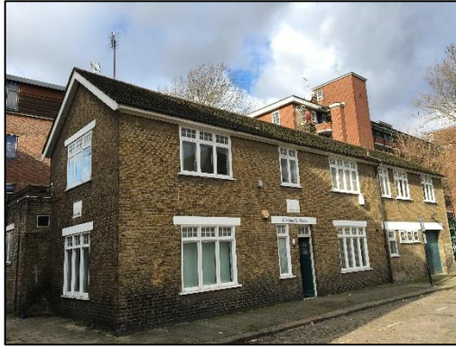
Figure 1: Two-storey section viewed from Ferdinand Place to the east
