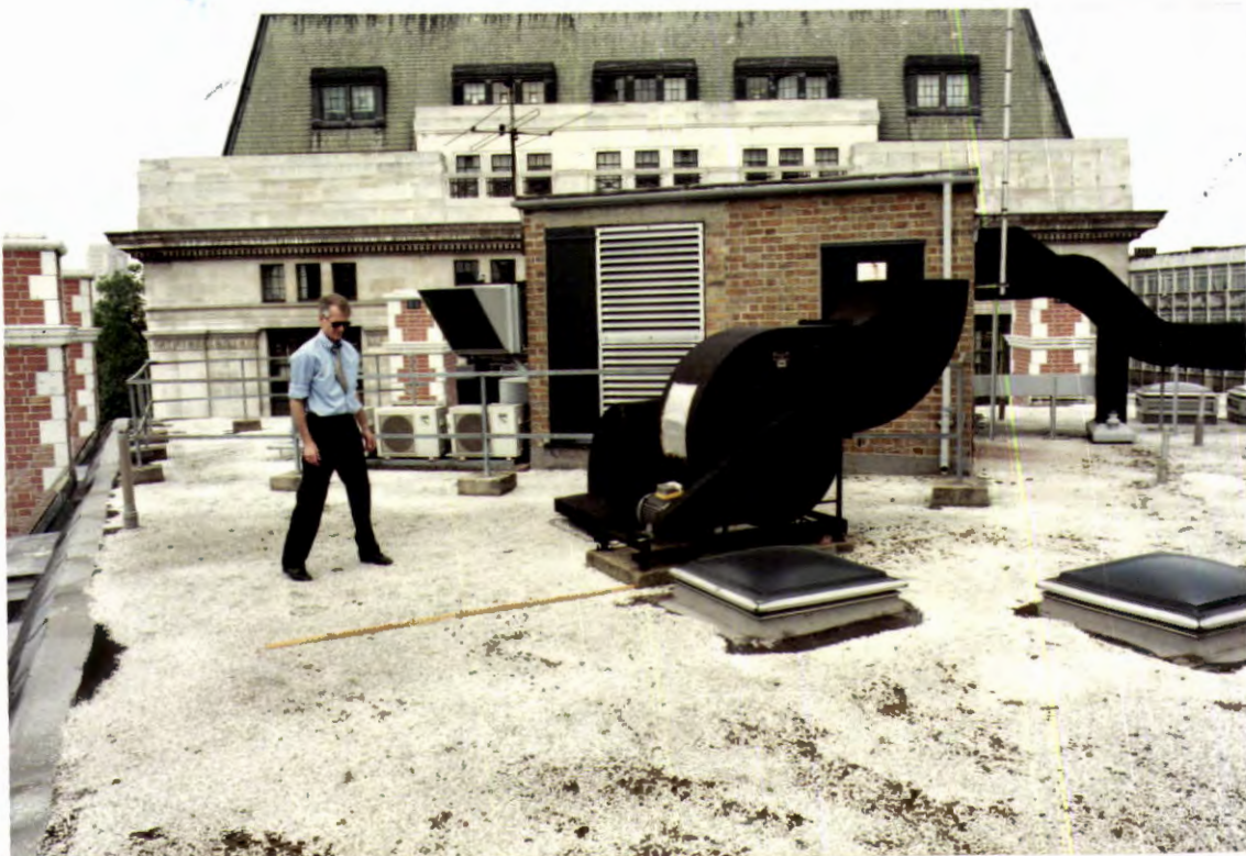
Roof - TOWARDS VERNON PLACE
