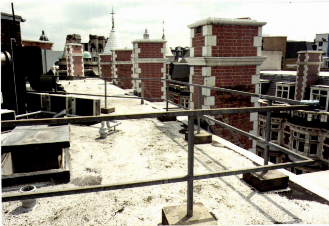
Roof - FROM VERNON PLACE / SICILIAN AVENUE. COX
