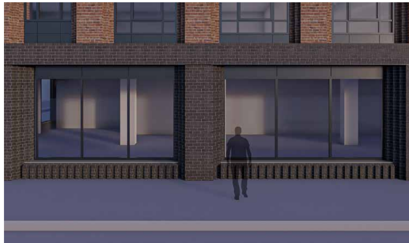
leicester blue brickwork piers between large office windows, with corbelled stall risers
