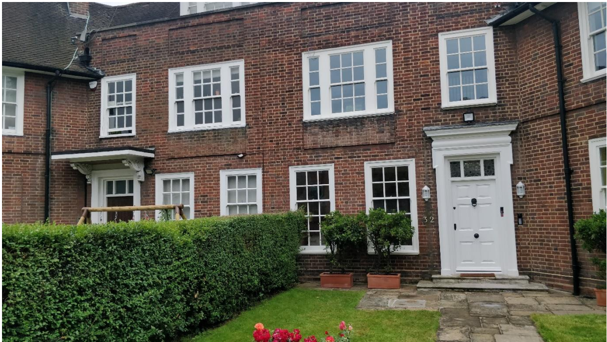
Above - Existing Front of 34 (Left) and 34 (Right) Ellerdale Road.
