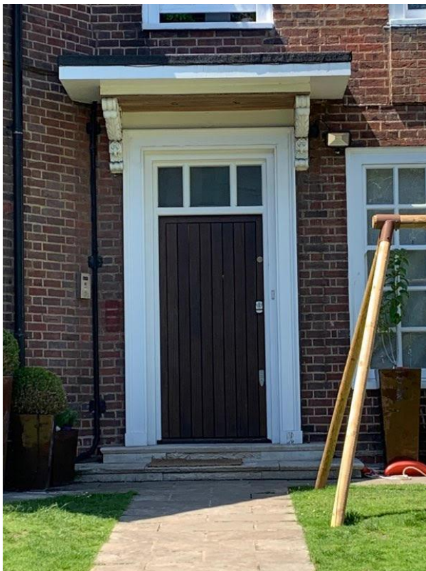
Above - Existing Front of 34 Ellerdale Road.
