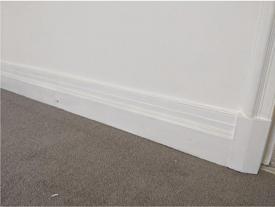
Figure 11: Third floor skirting
