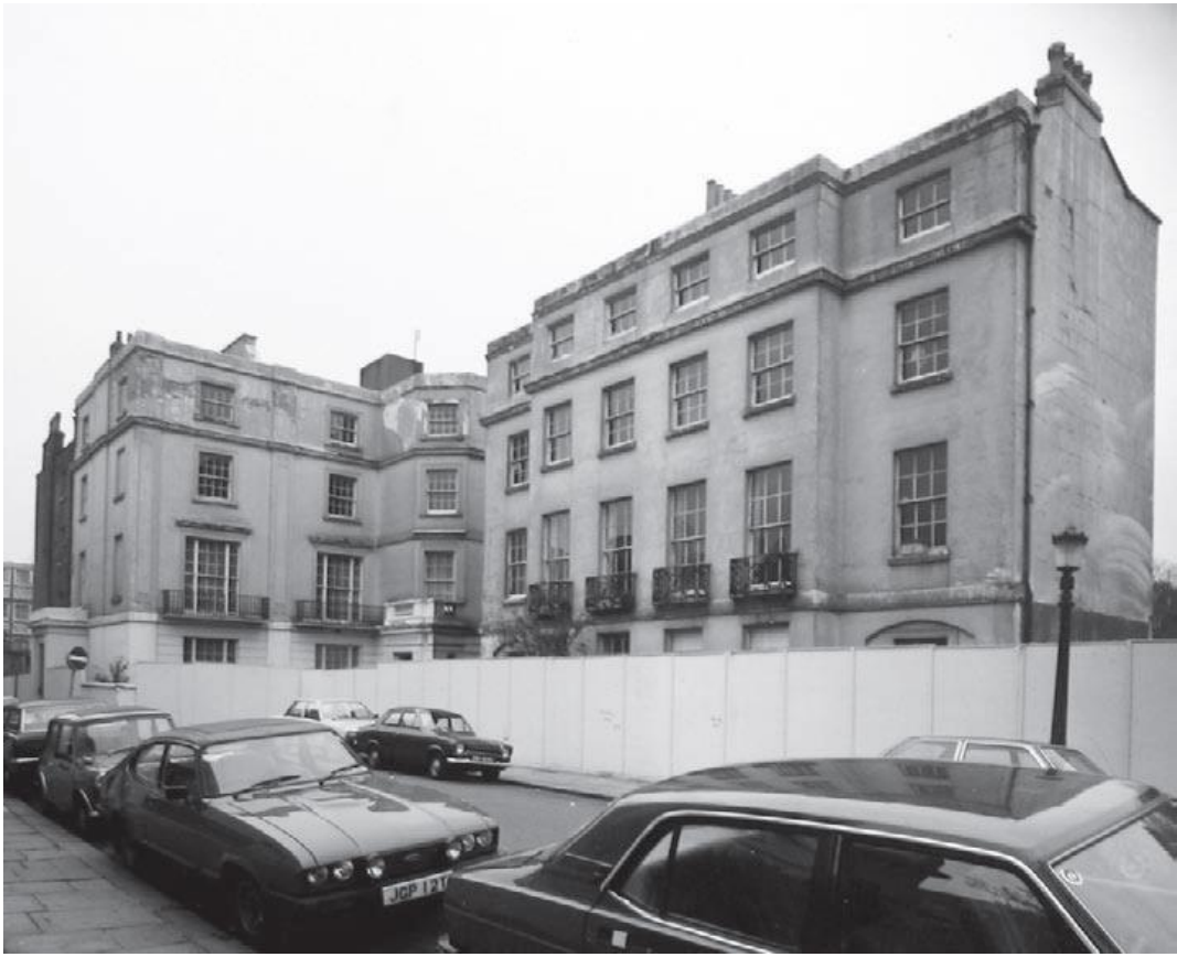
Figure 7: 1-2 Chester Gate before 1980's refurbishment
