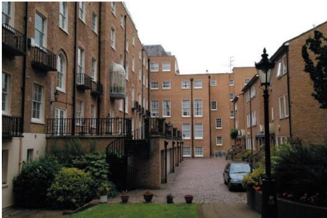
Figure 8: Rear courtyard of Chester Gate looking north
