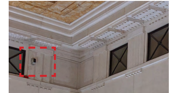
Existing Smoke detectors where power could be supplied to luminaire
