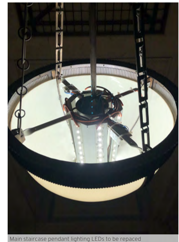
Main staircase pendant lighting LEDs to be repaced
