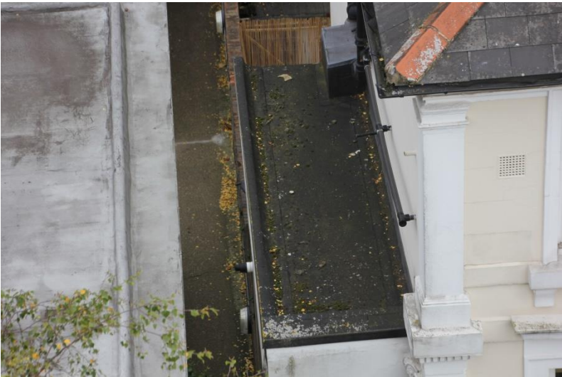
Photo 7. No. 6 Oak Court - flank flat roof
