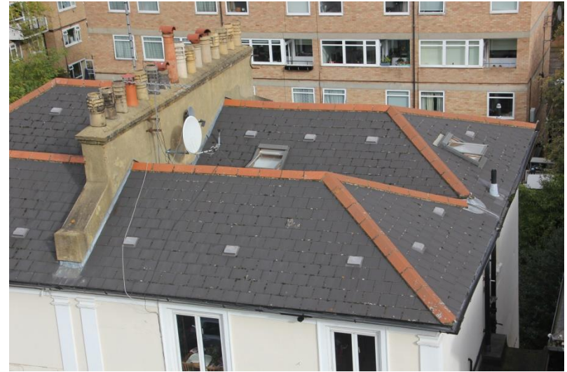
Photo 10. No.3 Oak Court - main roof
