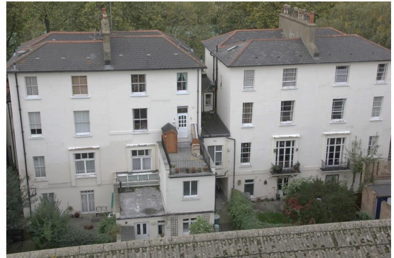
Photo 4. Nos.3-6 Oak Court - rear elevations
