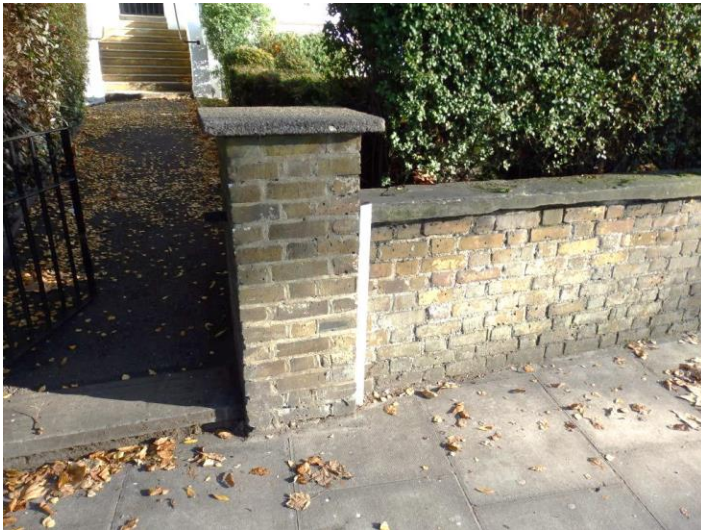
Photo 15. Oak Court - front boundary wall
