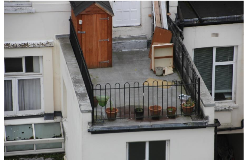
Photo 6. No. 4 Oak Court - higher level flat roof
