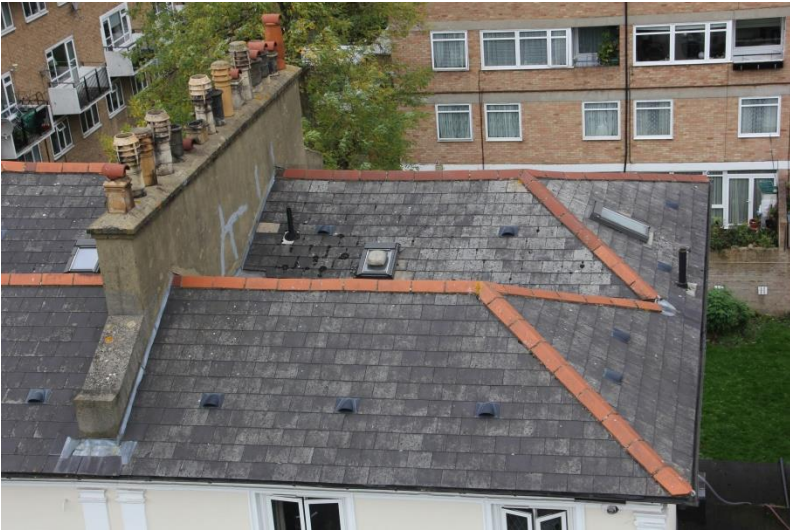
Photo 9. No. 5 Oak Court - main roof
