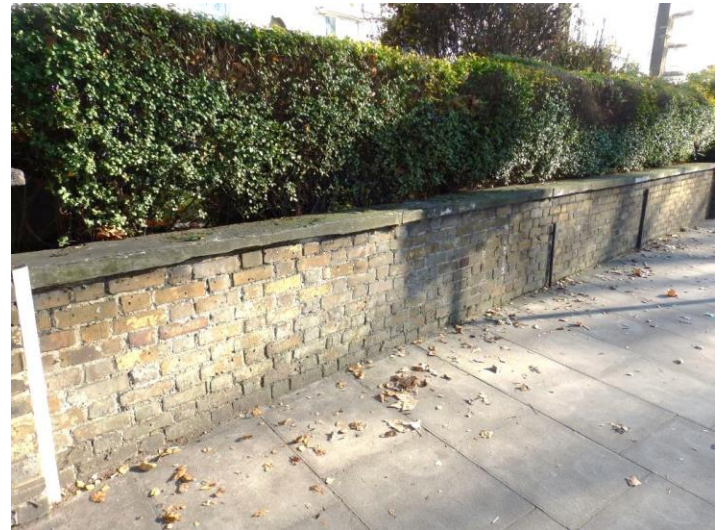
Photo 16. Oak Court - front boundary wall
