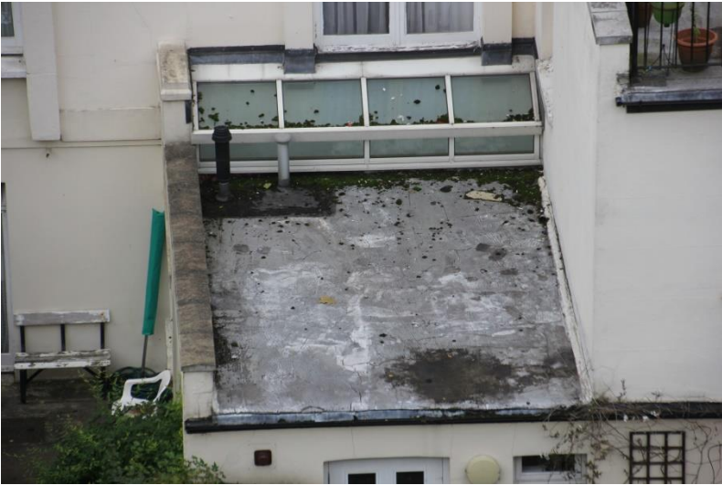
Photo 5. No. 4 Oak Court - lower flat roof
