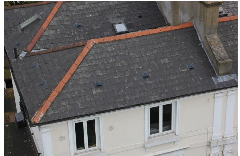
Photo 8. No.6 Oak Court -main roof
