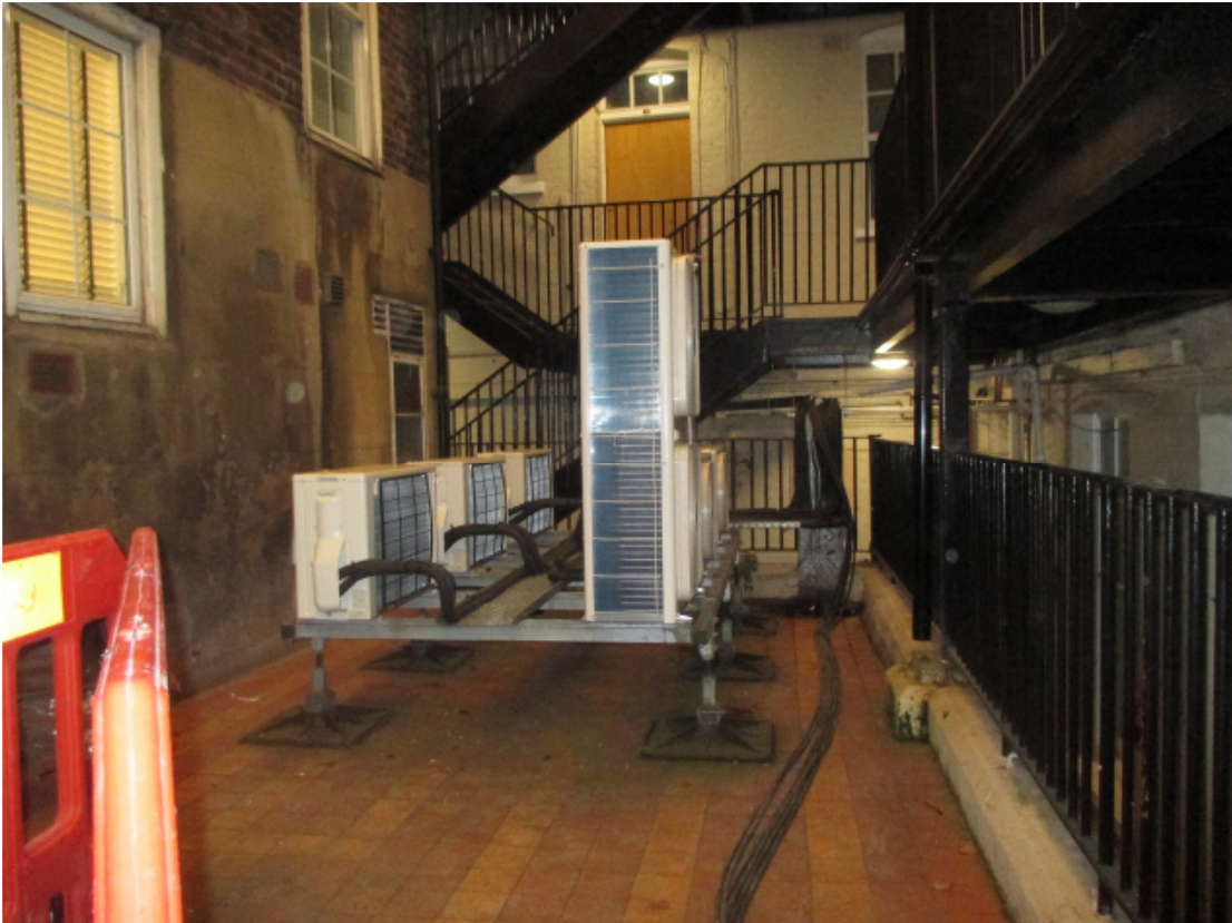
4. View towards side of existing a/c units
