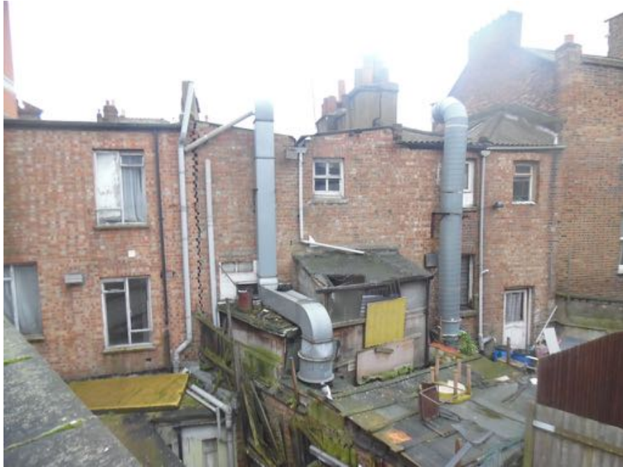
PH1 - Rear view of no.s 3, 5 & 7
