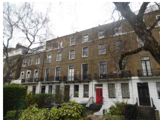
PH22 - View of 4 storey Georgian residential terrace
