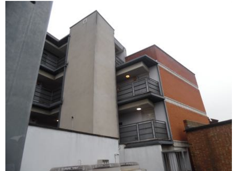
PH10- View of no.s 1-34's walkways & lift shaft
