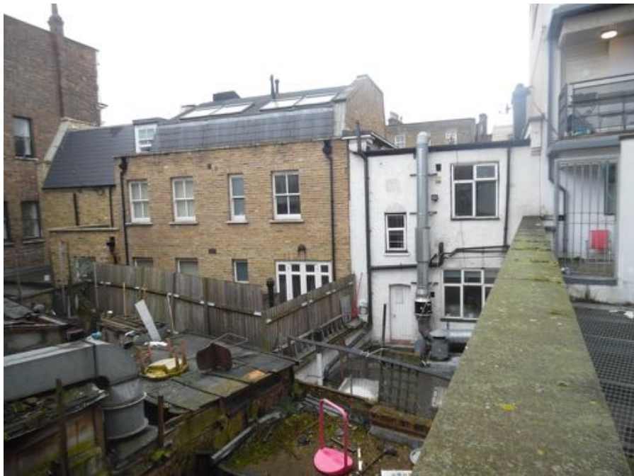
PH3 - Rear view of no.s 4, 6 & 8
