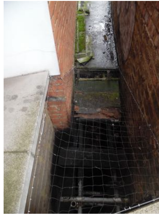
PH7 - View down of no.7 & 1-34's gap
