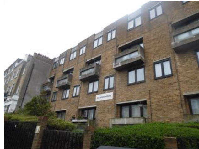
PH20 - View of Modern apartment block
