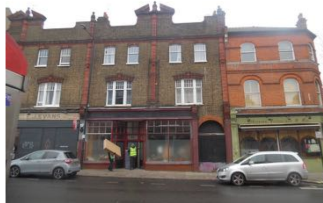
PH15 - View of nos 12, 14 & 16
