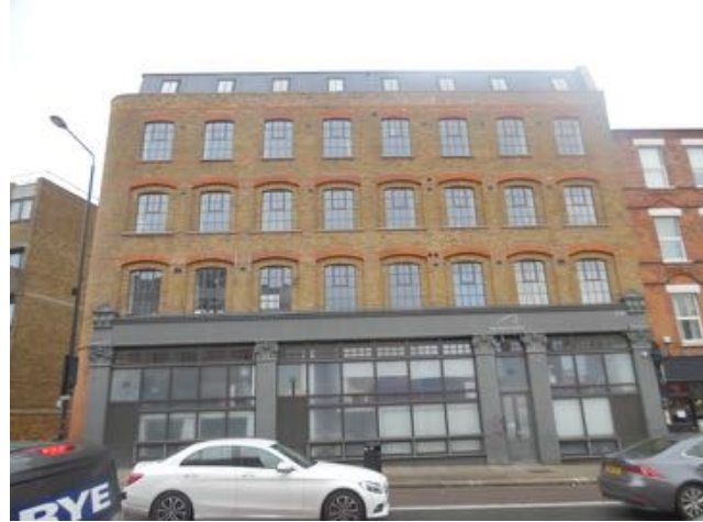
PH17 - View of no.s 28 to 34
