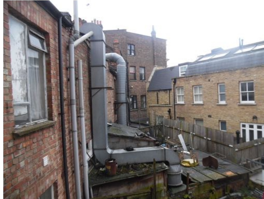
PH2 – View of no.s 4, 6 & 2
