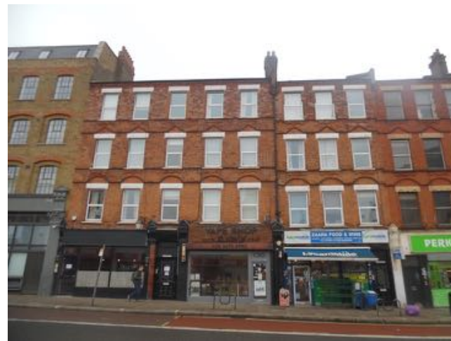
PH16 - View of nos 18, 20 & 22
