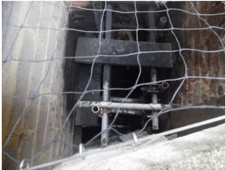
PH8 - View down of no.7 & 1-34's gap
