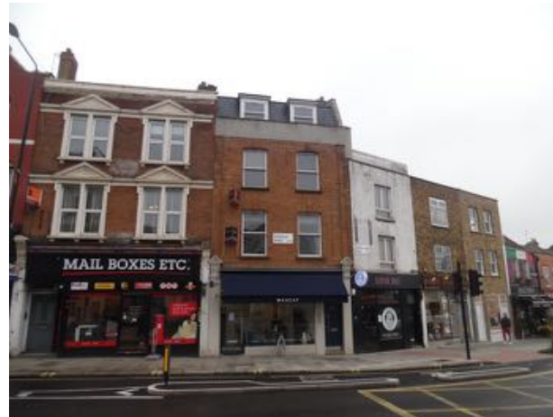
PH11 - View of no.s 4, 326 & 324
