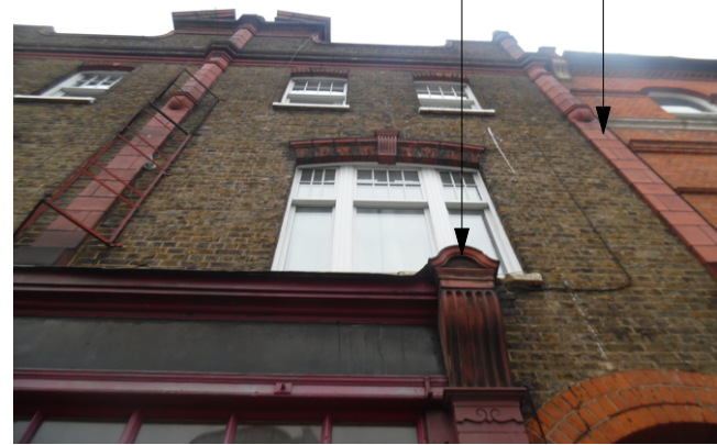
Photo of no.6 Fortess Road
