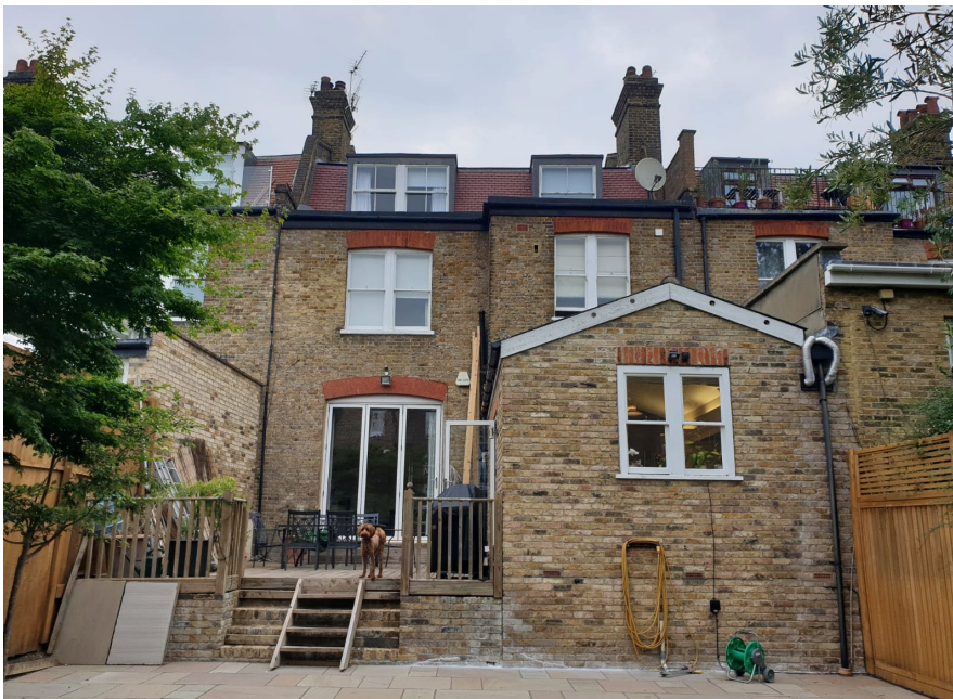
Photograph of Rear Elevation
