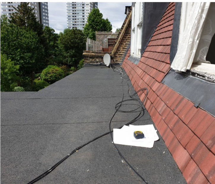
Below Right: Terrace/Balcony at 217
