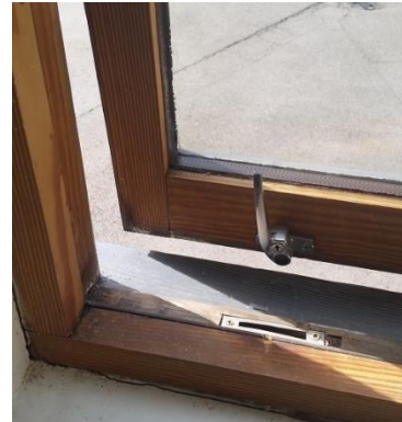
Example of a window opening impeded by reveal
