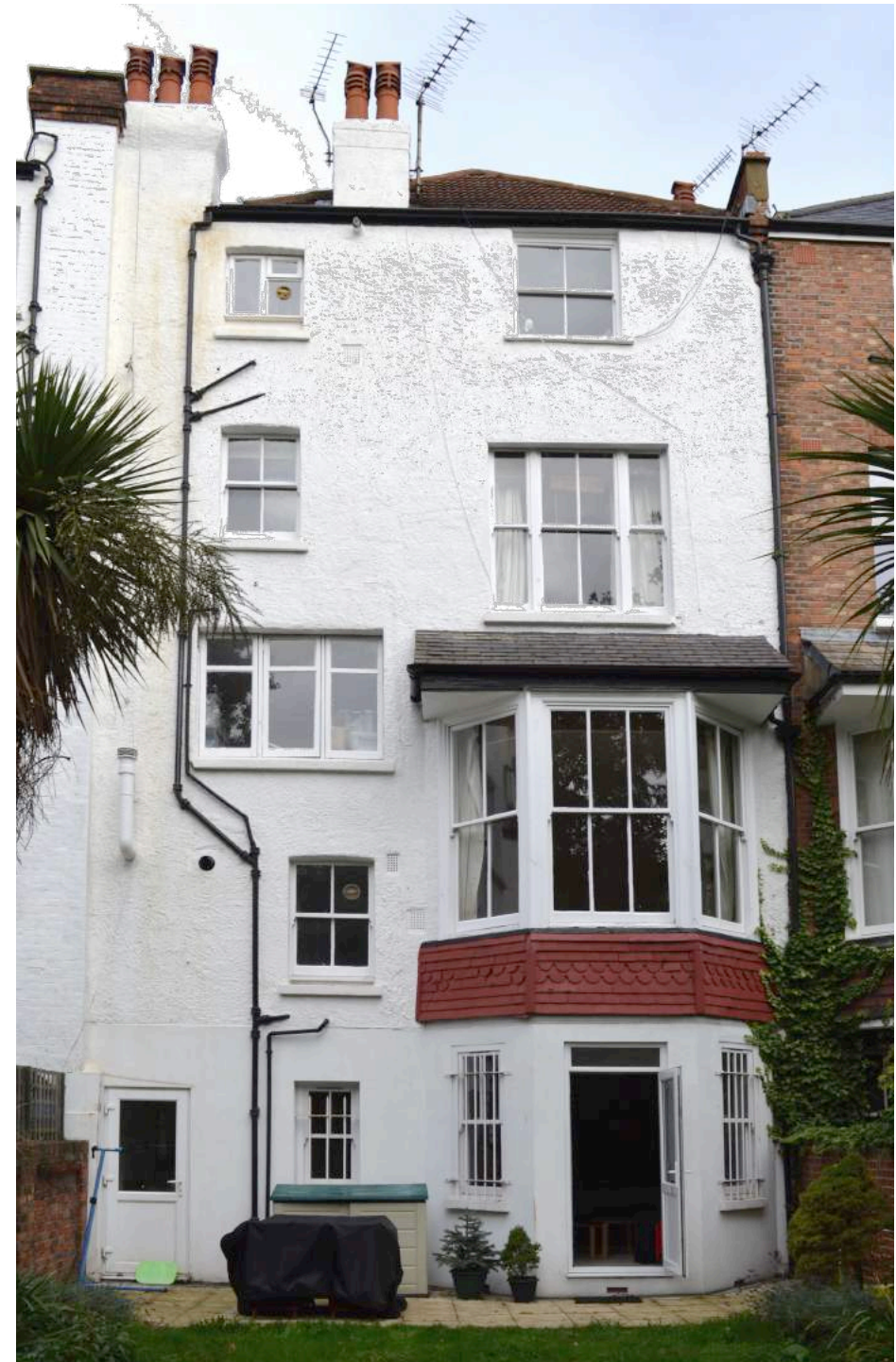
B Existing Rear Elevation Photograph
