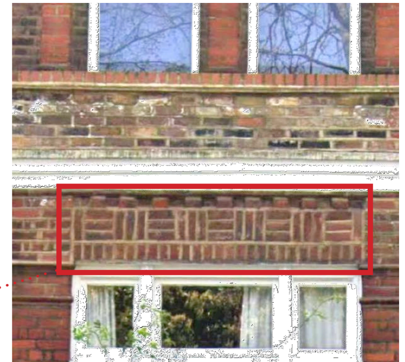
▲ Fig 21. Front elevation decorative brickwork - Broadhurst Gardens
