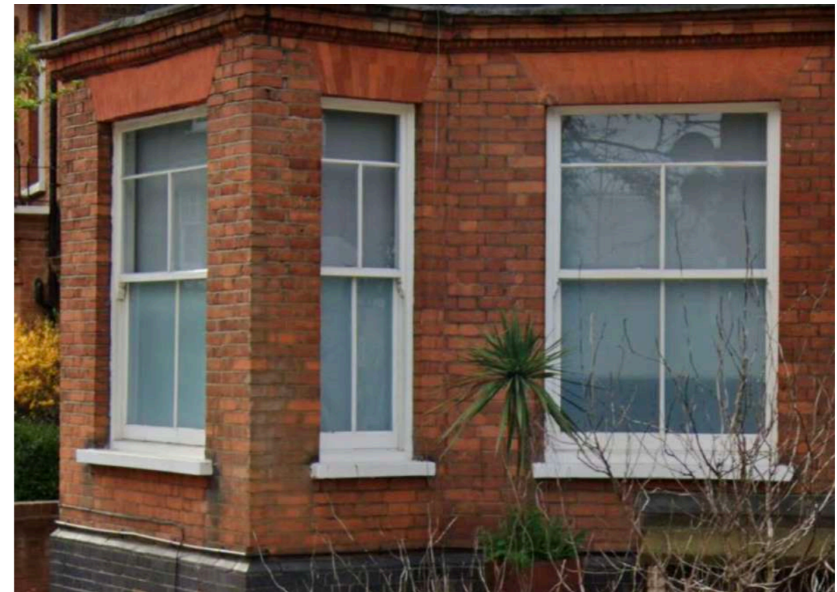
▲ Fig 26. Example of proposed sash windows from elsewhere in the South Hampstead conservation area
