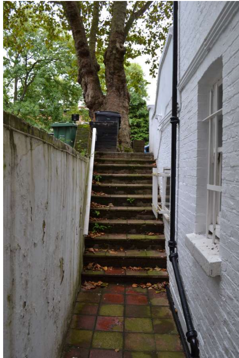
▲ Fig 30. Existing front entrance
