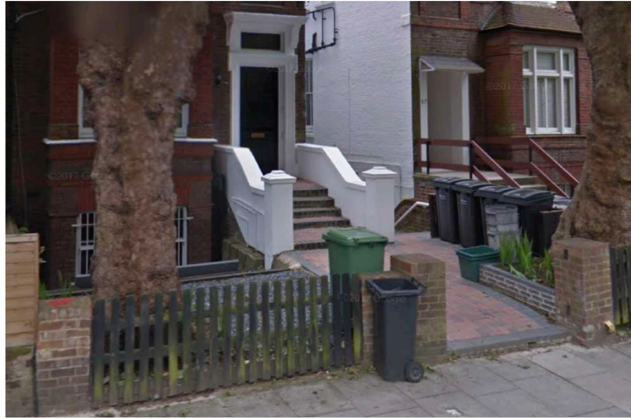
▲ Fig 9. Front entrance view from street 01
