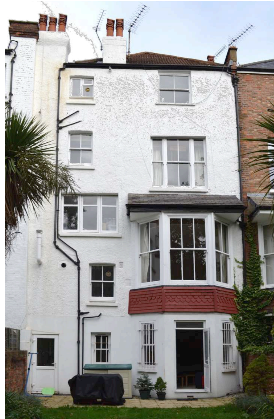
B Existing Rear Elevation Photograph
