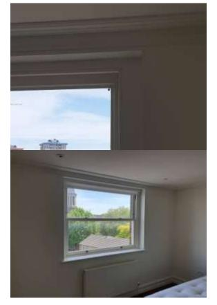
W3.05 Stairwell Rear Slimlite Double Glazed upper Double glazed Alum spacer bottom
