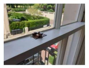
W1.02 / W1.03 Internal view Master Bed All windows in good condition Evidence of previous refurbishment including insertion of brush draught proofing and replacement glass.
