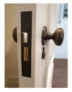
DG.01 Front door – internal Original – good condition. Minor repairs/redec only.
