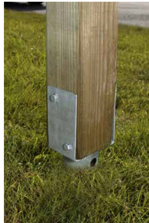
TYPICAL PLAYHOUSE POST SUPPORT INSTALLED
