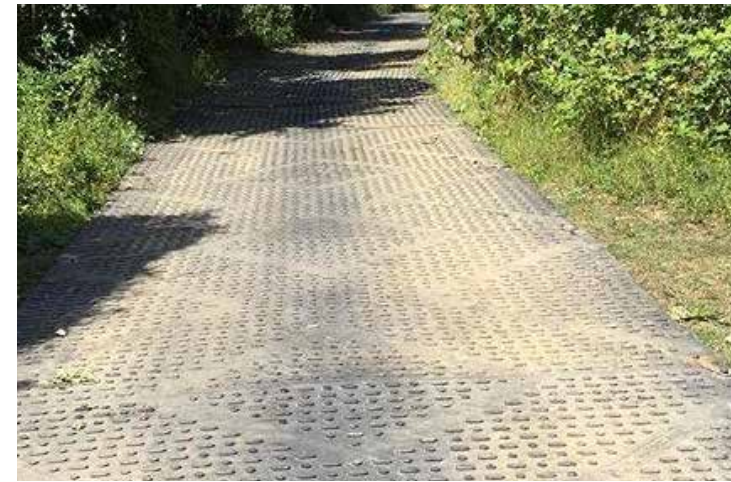
A. Temporary ground protection (if wet)
