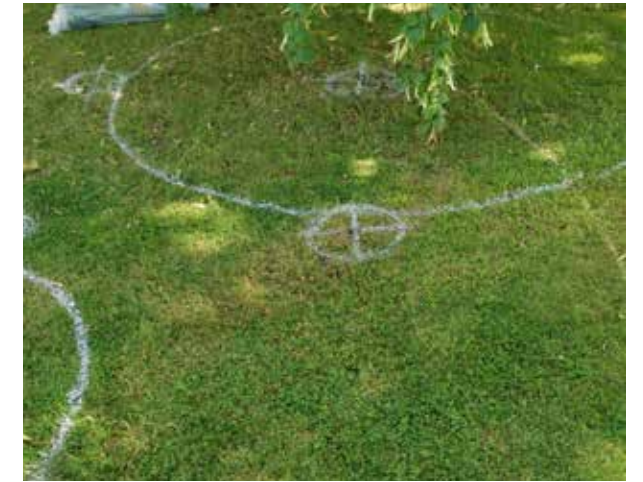
B. Setting out ground screw locations
