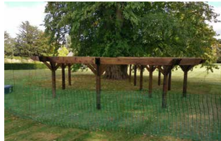
C. Erection of Playhouse platform
