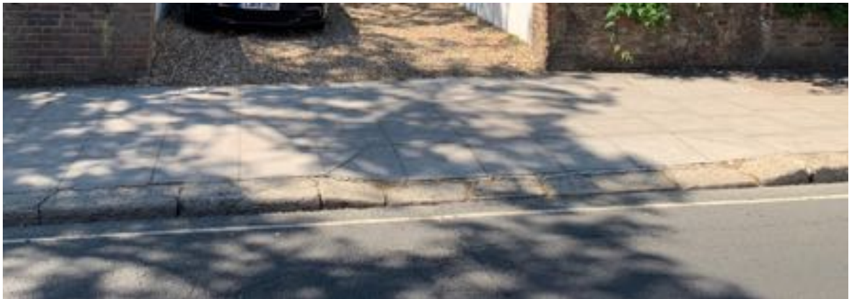
Current photo showing the misalignment of the dropped kerb and the brick piers at the entrance to 131 Haverstock Hill
