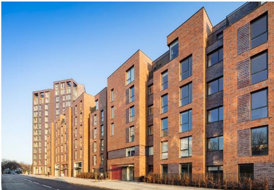
Figure 4: An image of the completed Phase 1 scheme.
