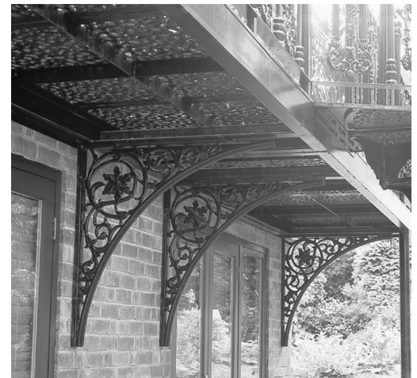
EXAMPLE OF BALCONY IRON BRACKETS
