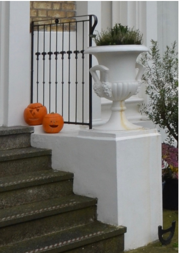
Existing front door railings design to be used for new railings. Terrazzo steps to be replaced with stone.
