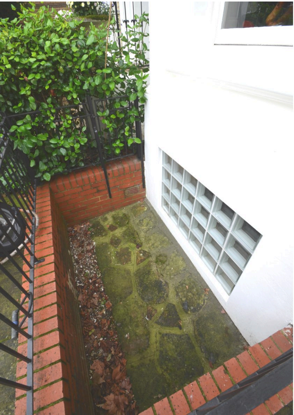
Existing: lightwell with glass bricks window.
