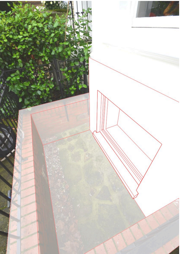
Proposed: lightwell base and window cill lowered. Walls rendered to match house. New painted timber window with stone cill.
