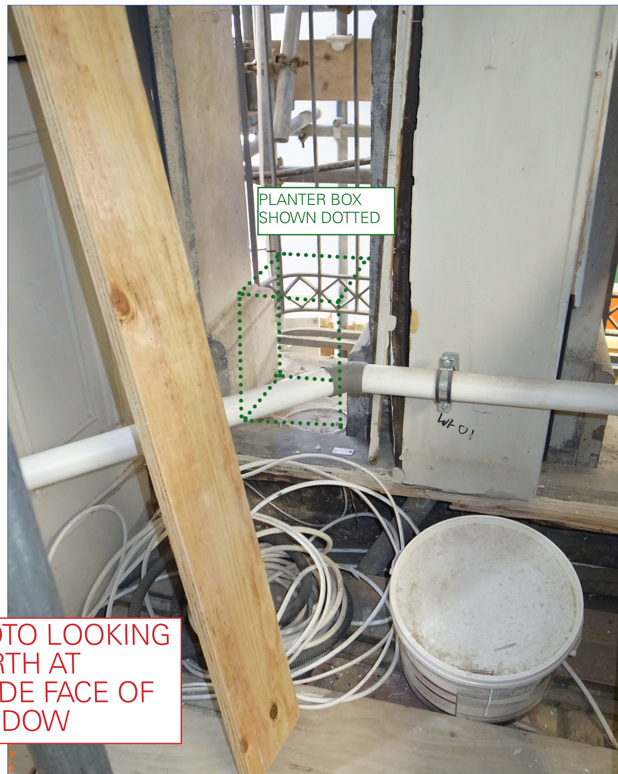
PROPOSED WIRING TO COME THROUGH 25MM WIDE NON-ORIGINAL MORTAR JOINT BETWEEN EXTERNAL STONE & TIMBER WINDOW FRAME
