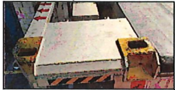
Hoist point roof
